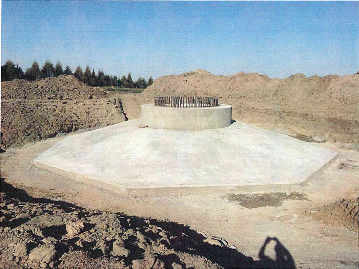
Complete Foundation at Turbine 1
