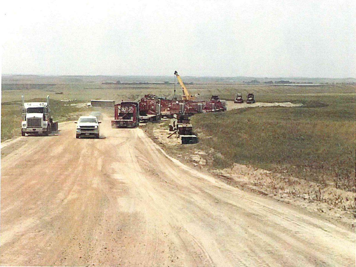
Crane Components Arriving Onsite
