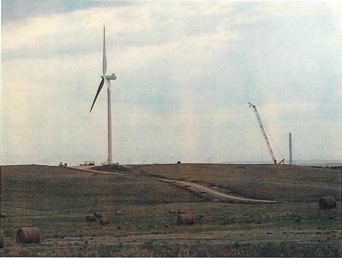
First Turbine Erected
