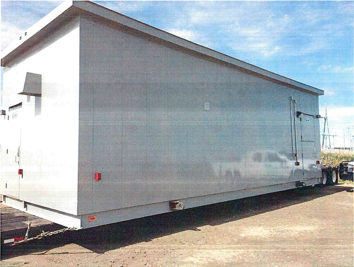
Substation Control Building Arrives Onsite
