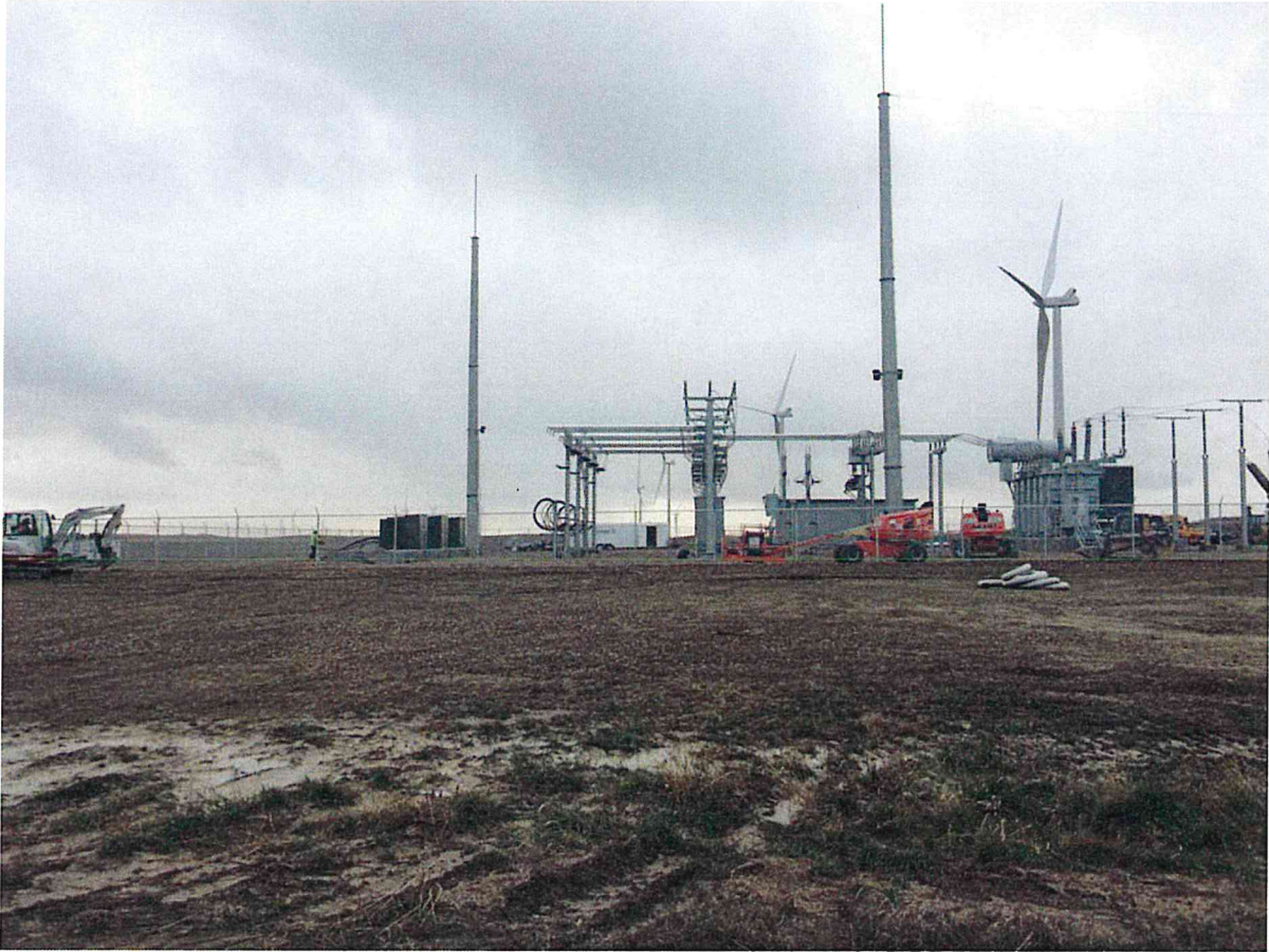
Substation Nearly Complete
