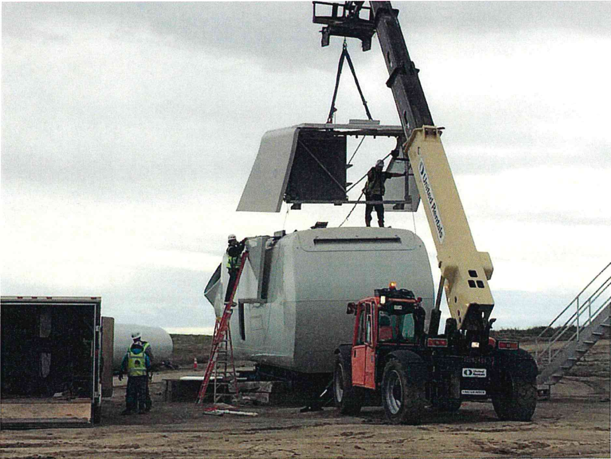
Installing Cooler Top on Nacelle
