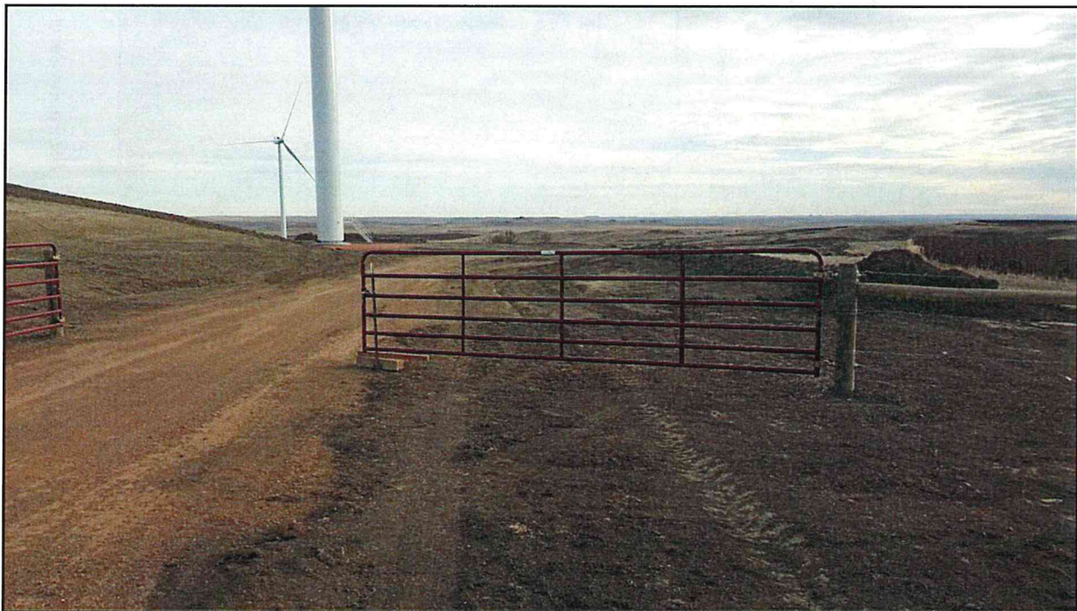
Figure 6. Gates were installed at the intersections with existing fence lines.
