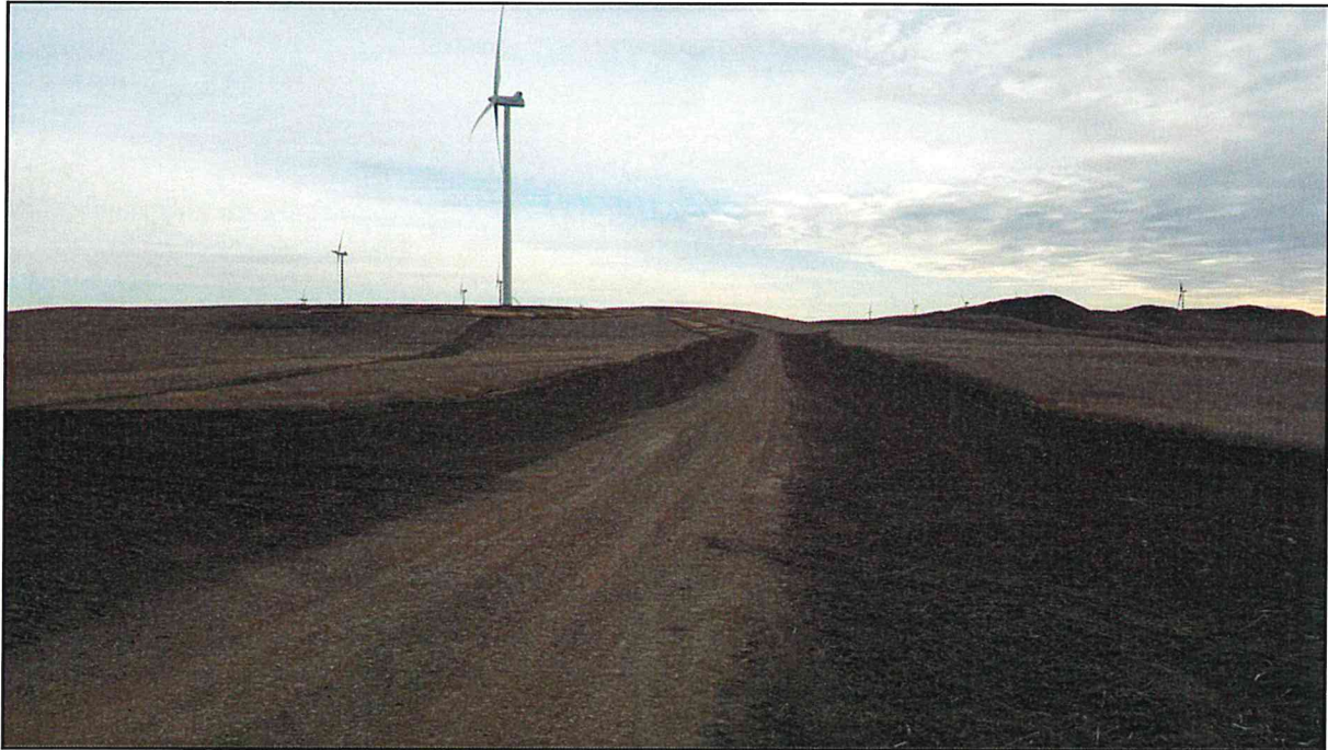
Figure 1. Photo of reclaimed access road between T1 and T2. Seeding was complete where grasslands were adjacent to the ROW.
