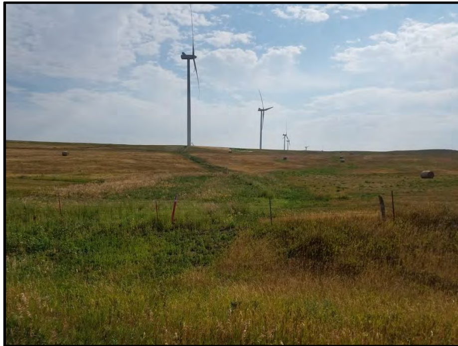
Photograph 2. View looking east along the underground collection line located in the SW1/4 of Section 19, T139N, R90W. Turbines 09, 10, 11, 12 can be seen.
