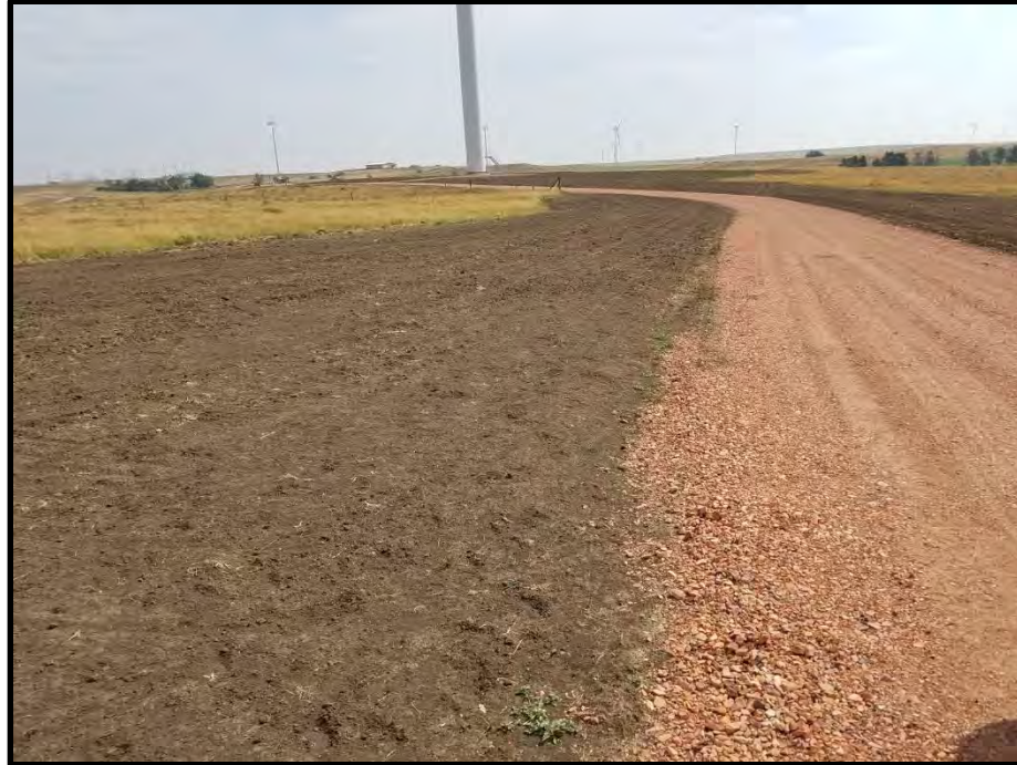
Photograph 3. View looking northeast along the access road in Section 30, T139N, R90W. Turbine 24 is nearest. Note the lack of vegetative growth in the disturbed area along the road.
