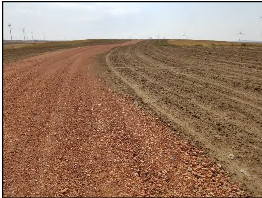
Photograph 4. View looking southwest along the access road in Section 30, T139N, R90W.
