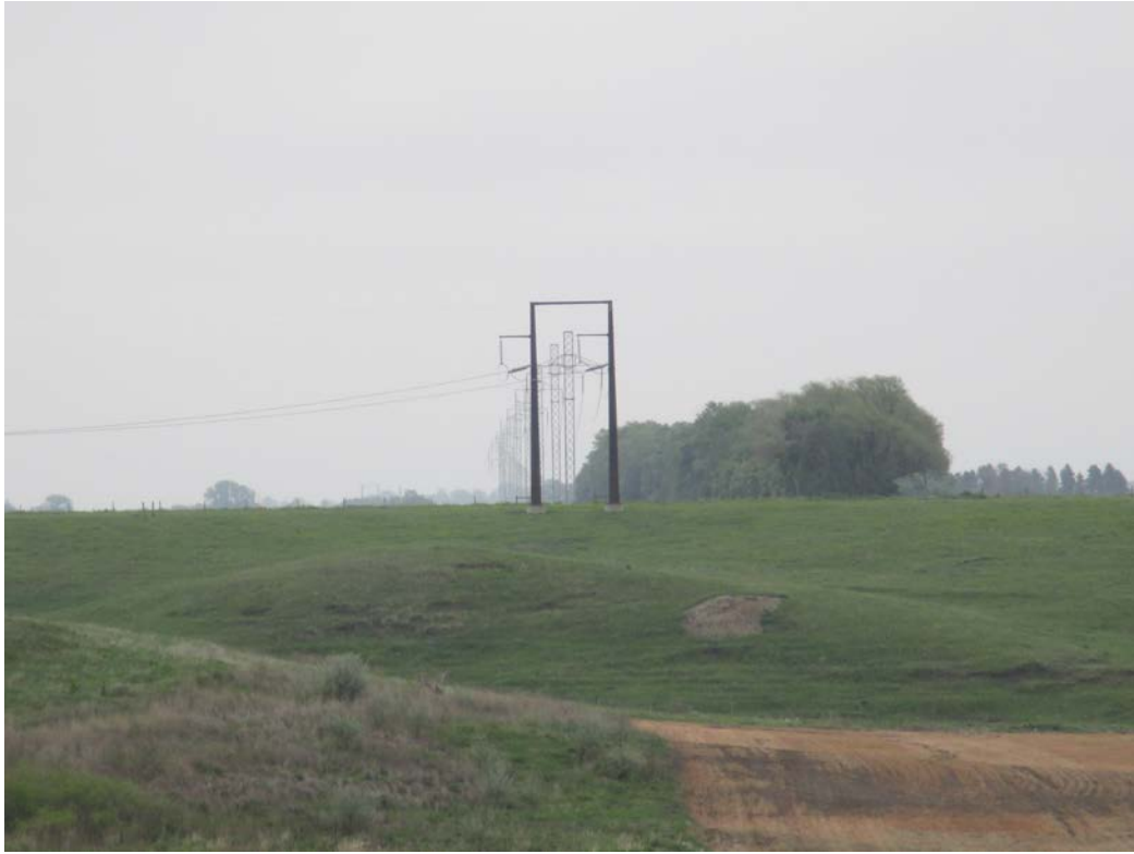
Above: Photo 5 (Near structure 1395) – Disturbed soil area on east end of reroute. Observe the new structure and previous transmission line structures behind disturbed area. Unknown if soil disturbance is from old structure or something else. Looking east.
