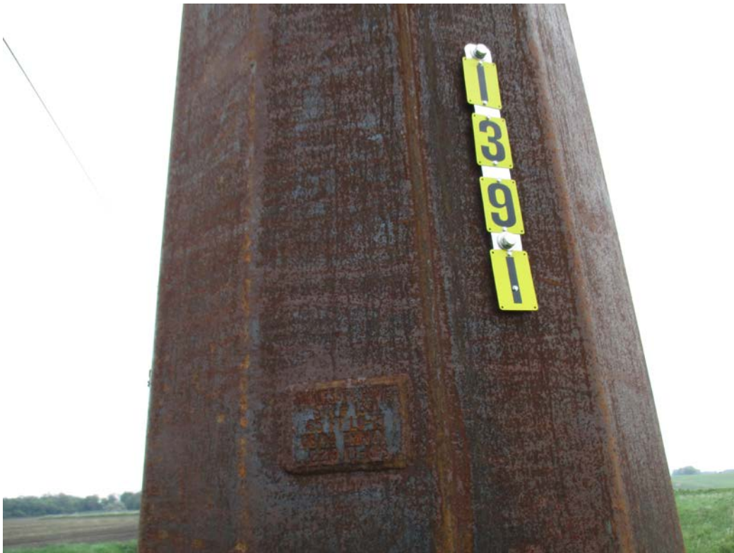
Below: Photo 2 (Structure 1391, Point 426) – Structure’s sign placards.
