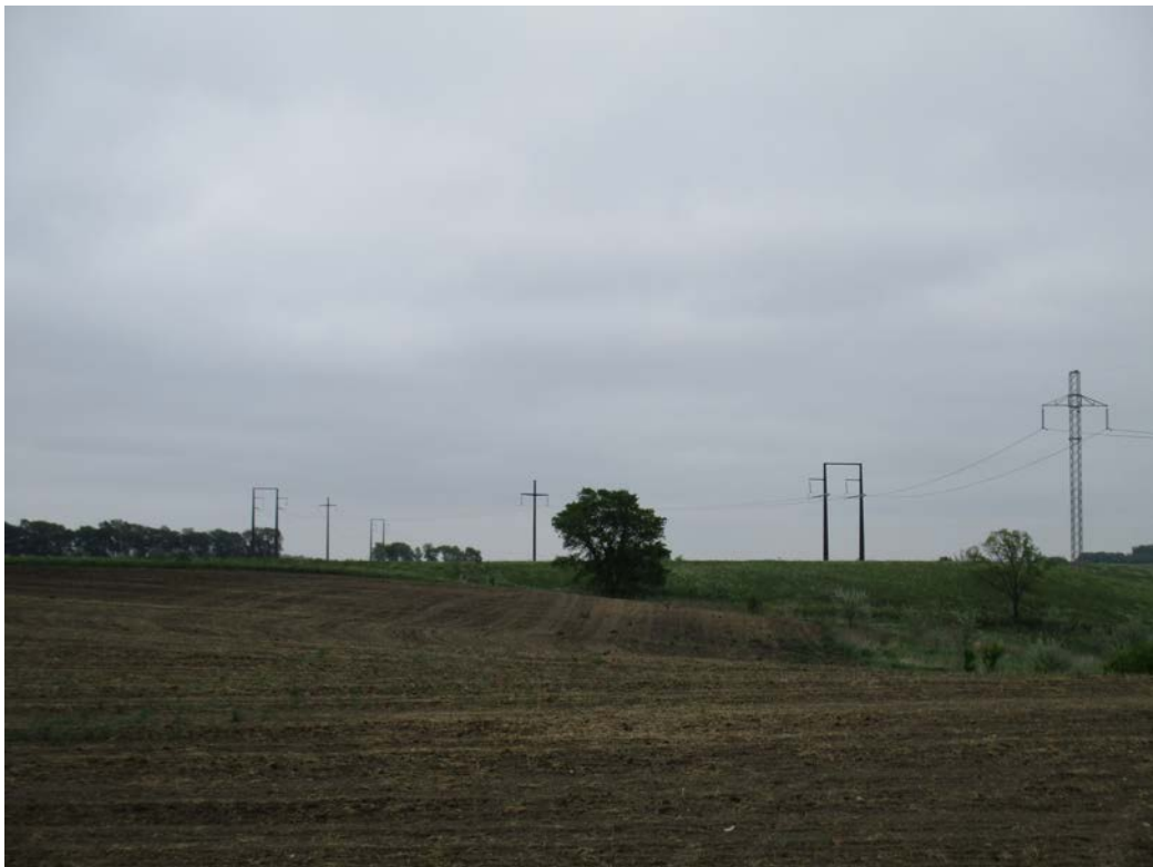
Below: Photo 14 – Overview of the area showing where the reroute connects to the existing transmission line (on the right). Looking east.
