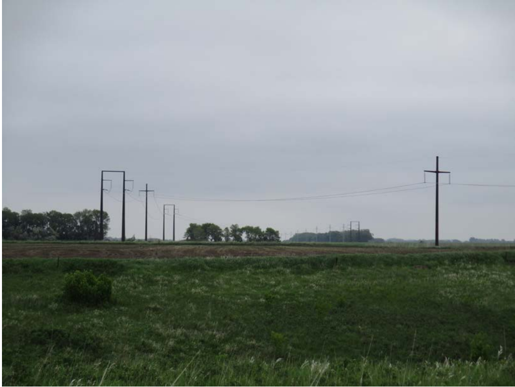
Above: Photo 13 – Overview of the area showing 5 of the 6 new rerouted transmission line structures.
