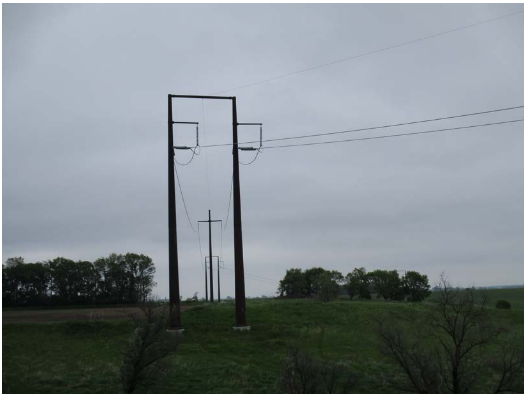
Below: Photo 8 (Structure 1391B, Point 429) – Transmission line structures going through a tree row. Looking east.
