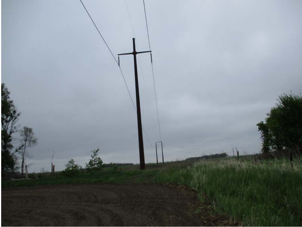
Above: Photo 9 (Structure 1391C, Point 430) – Single pole structure near tree row and recently planted agricultural field.
