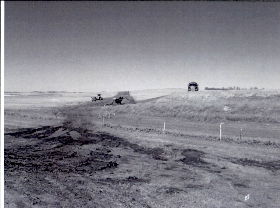
Photo 4: Recently completing boring and open trenched areas, awaiting reclamation / restoration activities.
