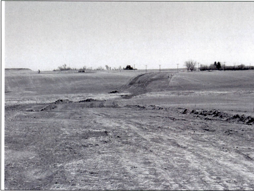
Photo 5: Stream boring area.
