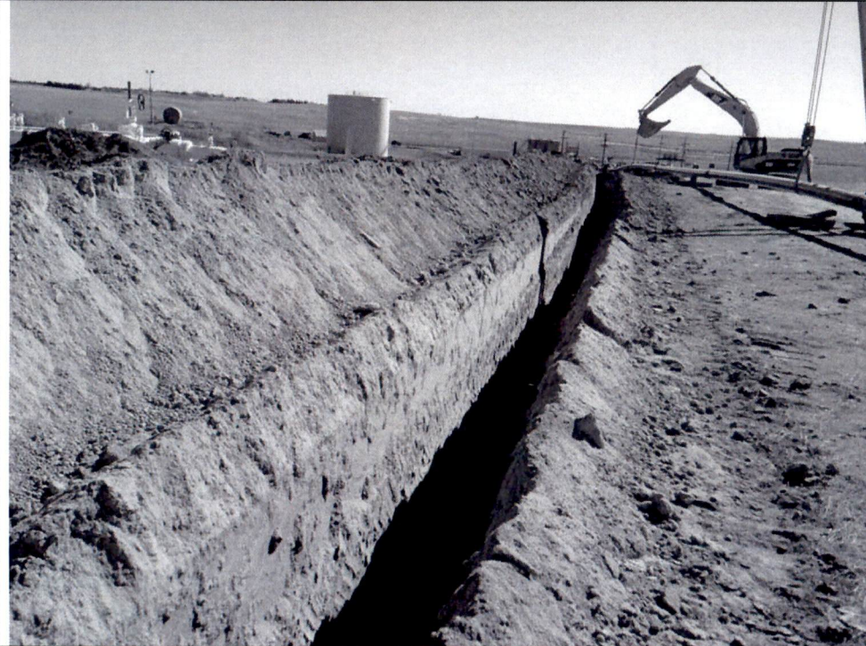
Photo 2: Active trenching areas and topsoil separation (background)
