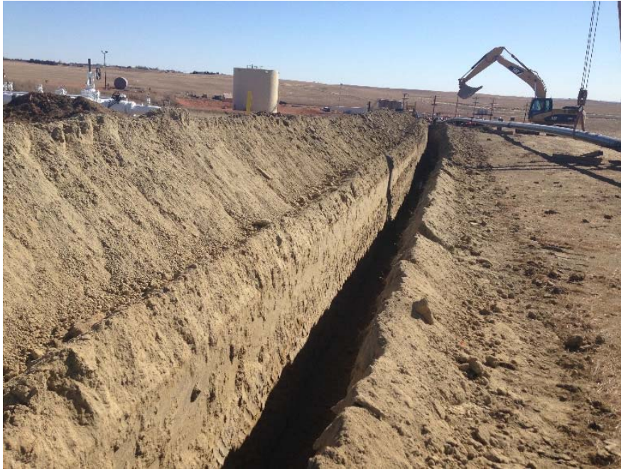
Photo 15: 3- During construction burial depths were visually confirmed.
