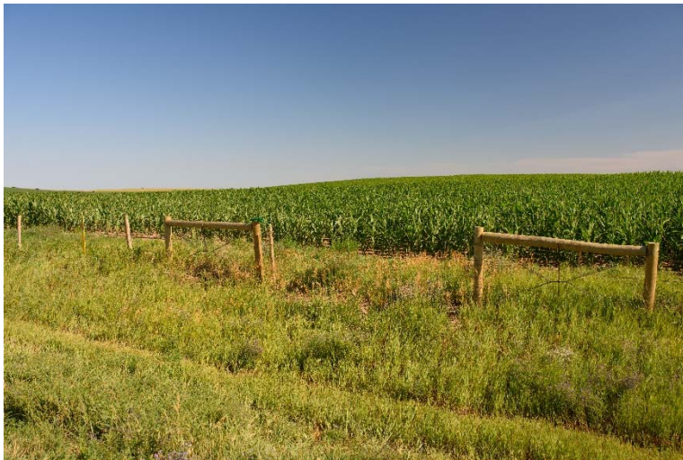
Photo 12: Installed fence repair and gate (facing Southeast).
