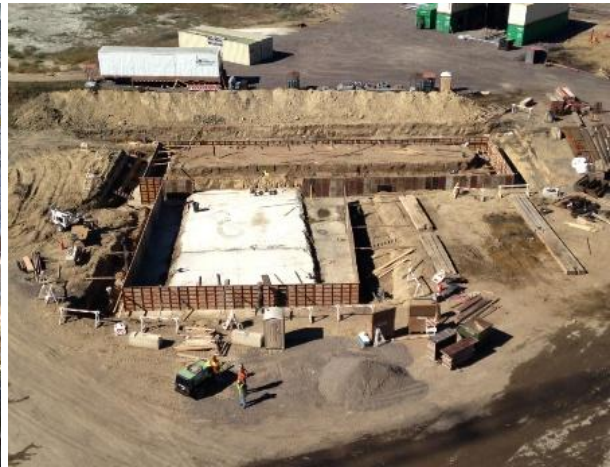
10-01 Ammonia foundation formwork
