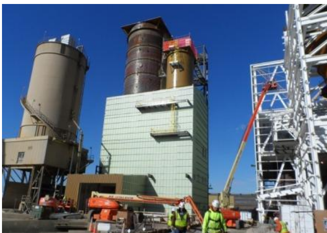
11-07 WA/PL liner panel installation
