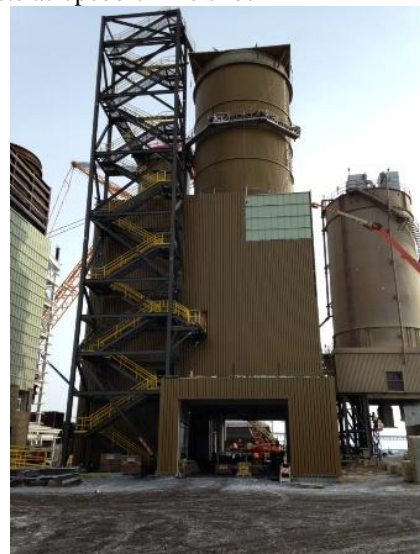
12-11 Siding work almost finished WA/PL
