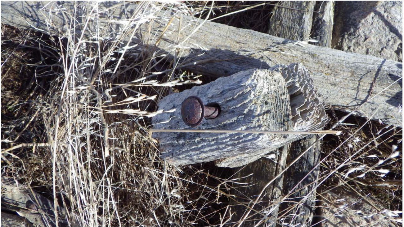
Figure 5: Close-up view of the handmade bolts in 32MZx1385 (Image 603).
