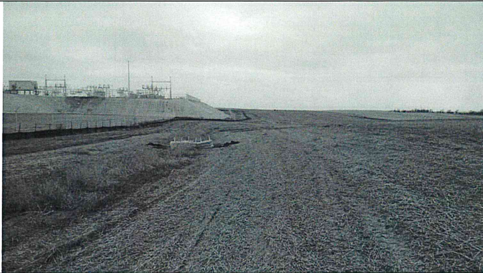
Photo 1: Downstream extent of project, showing erosion control measures.
