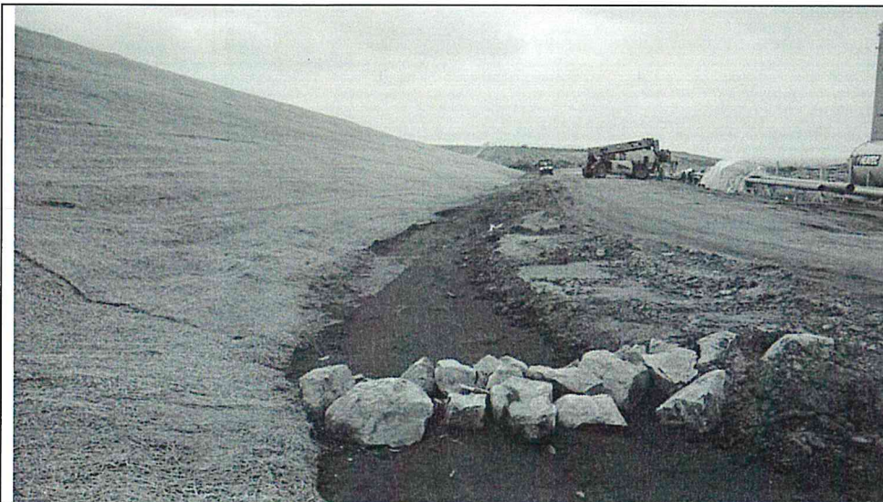
Photo 4: Rock checks in interior drainage ditch.
