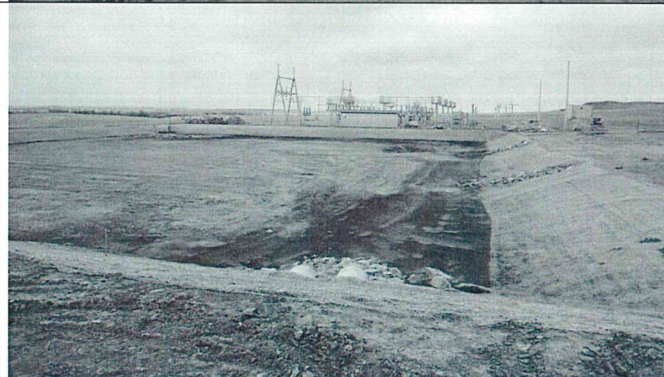
Photo 6: Stormwater pond, which will receive interior drainage, and provide spill containment onsite during operation.
