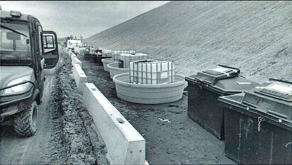
Photo 3: Barriers and secondary containment systems in place to prevent spills.
