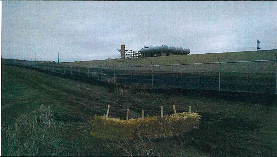
Photo 2: Looking upstream at silt fence and straw bales across the primary drainage from the onsite activities.
