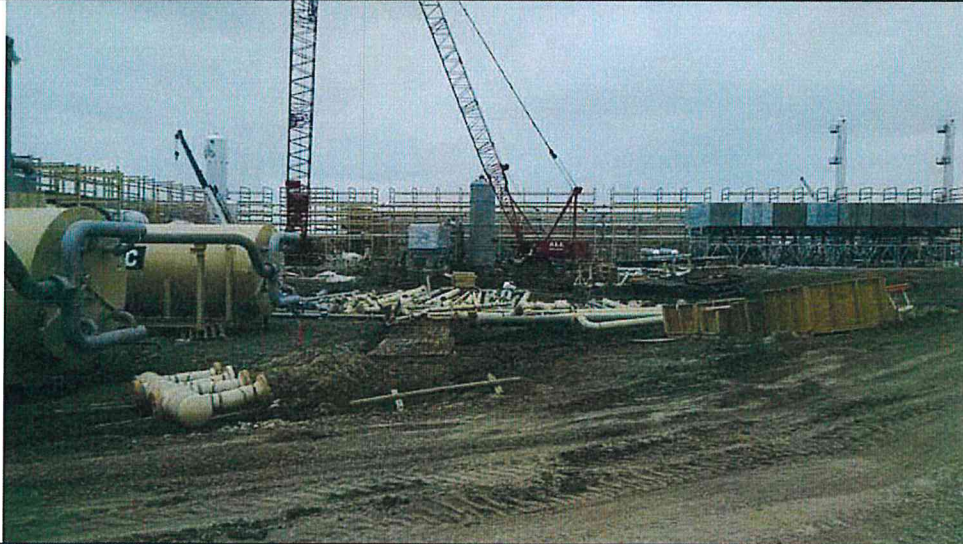
Photo 5: Interior construction area.
