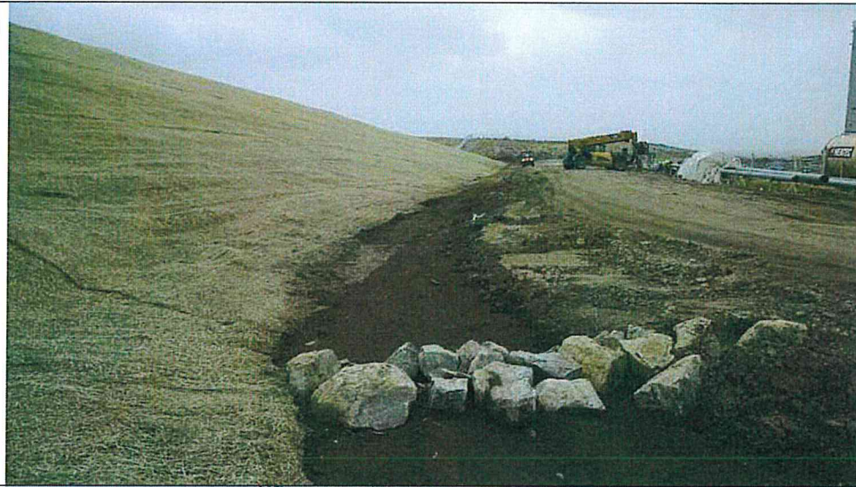
Photo 4: Rock checks in interior drainage ditch.
