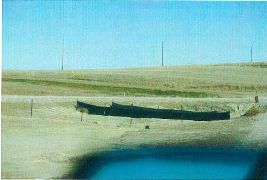
Photo 1: Entrance to facility, silt fence (facing northeast).
