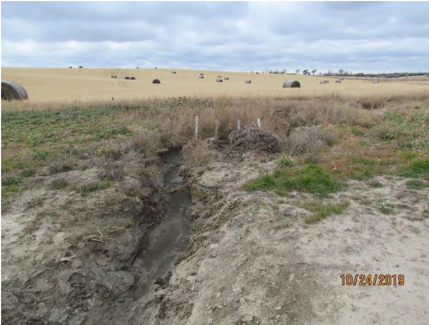
Photo 5: Gully formation at northwest portion of site.
