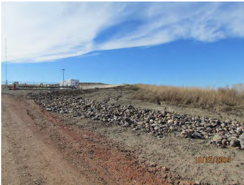
Photo 36: Facility road and ditch along southcentral portion of site 10-25-2019
