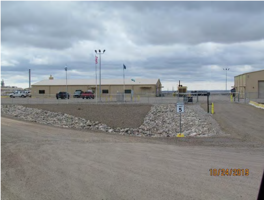
Photo 7: Lonesome Creek Gas Plant facility entrance 10-24-2019
