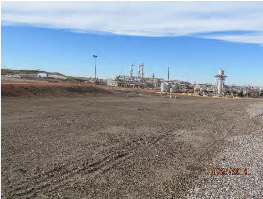
Photo 12: Inside the north portion of the facility.
