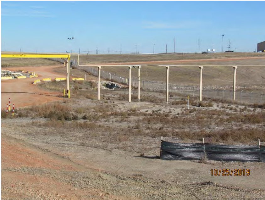
Photo 37: Silt fence and sparse vegetation at southeast portion of facility site 10-25-2019
