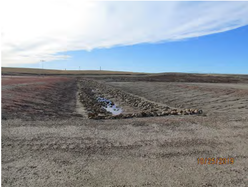
Photo 31: Stormwater conveyance ditch along southcentral portion of facility site 10-25-2019
