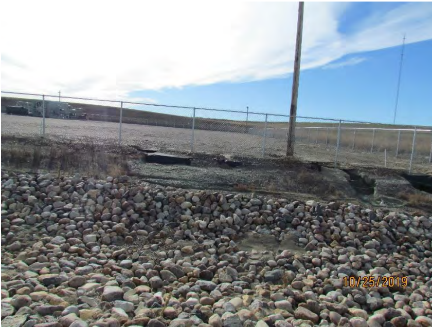
Photo 42: Stormwater conveyance path off southeastern fence line
