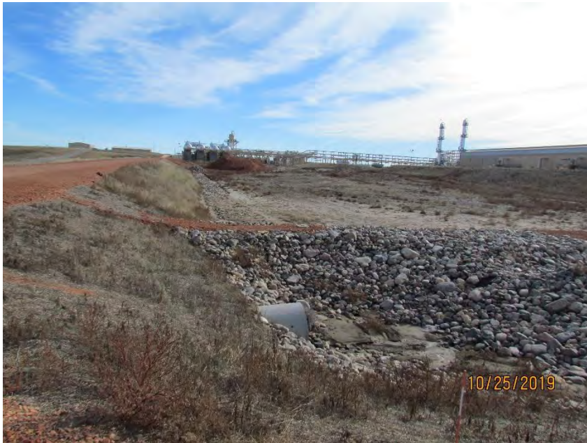
Photo 26: Facility road along northern extents of site, view of stormwater culvert
