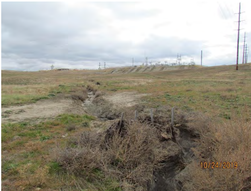
Photo 6: Gully formation at northwest portion of site.
