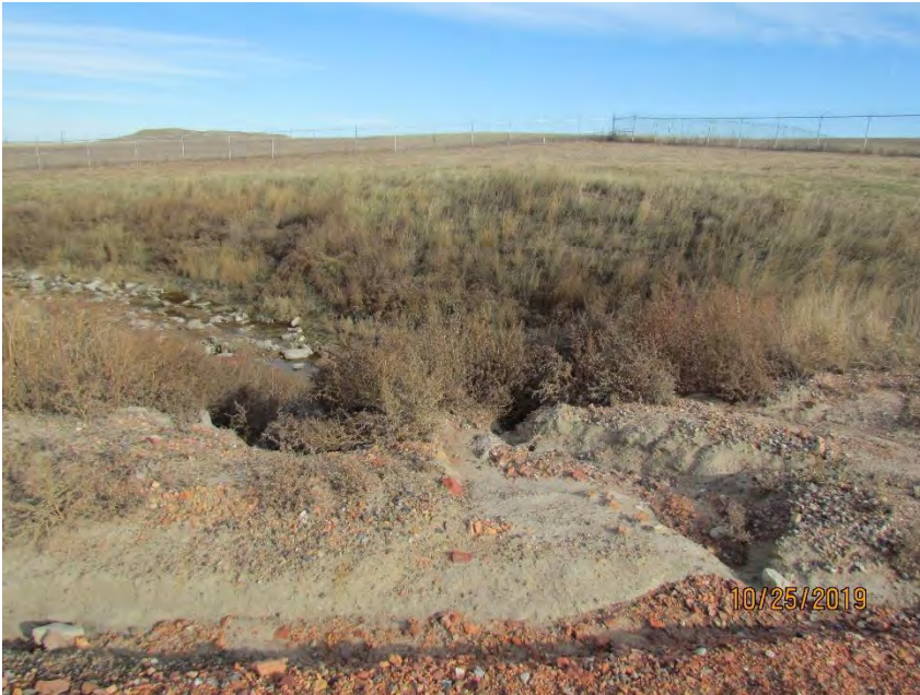
Photo 21: Gully erosion in northern extents of the facility
