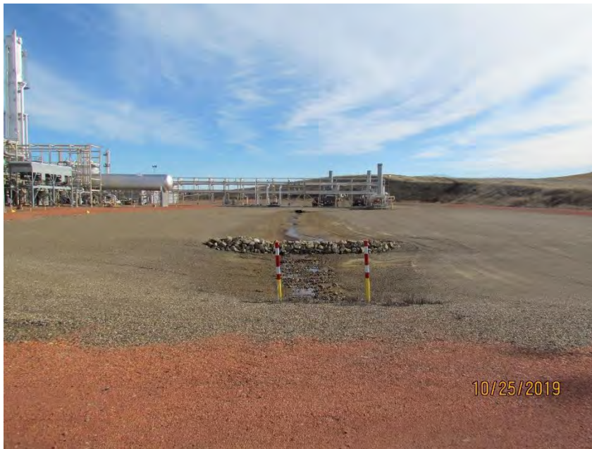
Photo 32: Southern extents of facility site, looking east at stormwater conveyance ditch 10-25-2019
