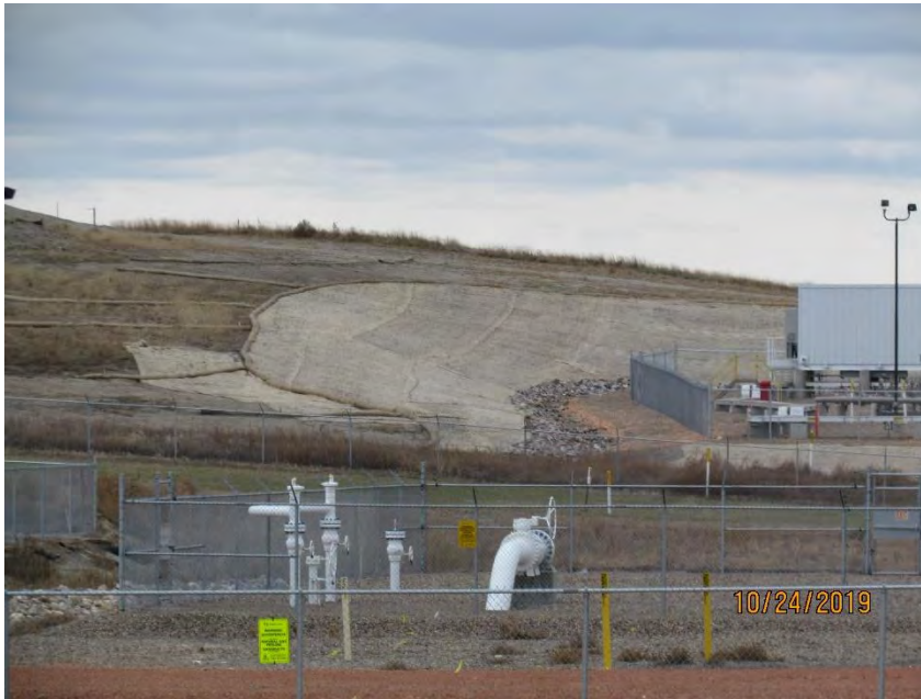
Photo 8: BMPs on slopes, east side of project site looking west 10-24-2019
