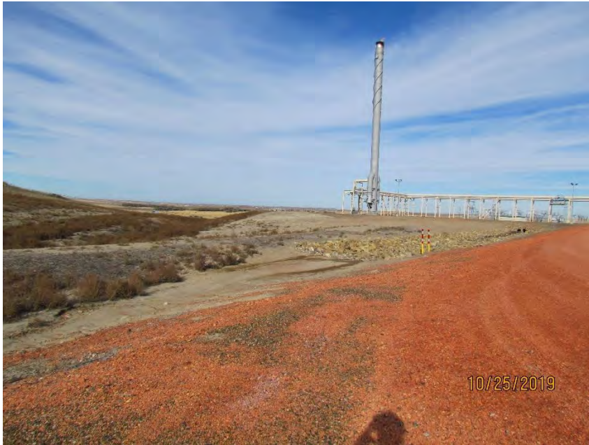
Photo 33: Southcentral side of the facility site looking northwest
