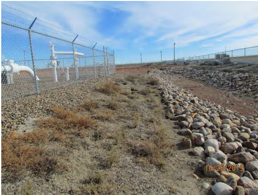
Photo 44: Southeastern extents of facility fence line
