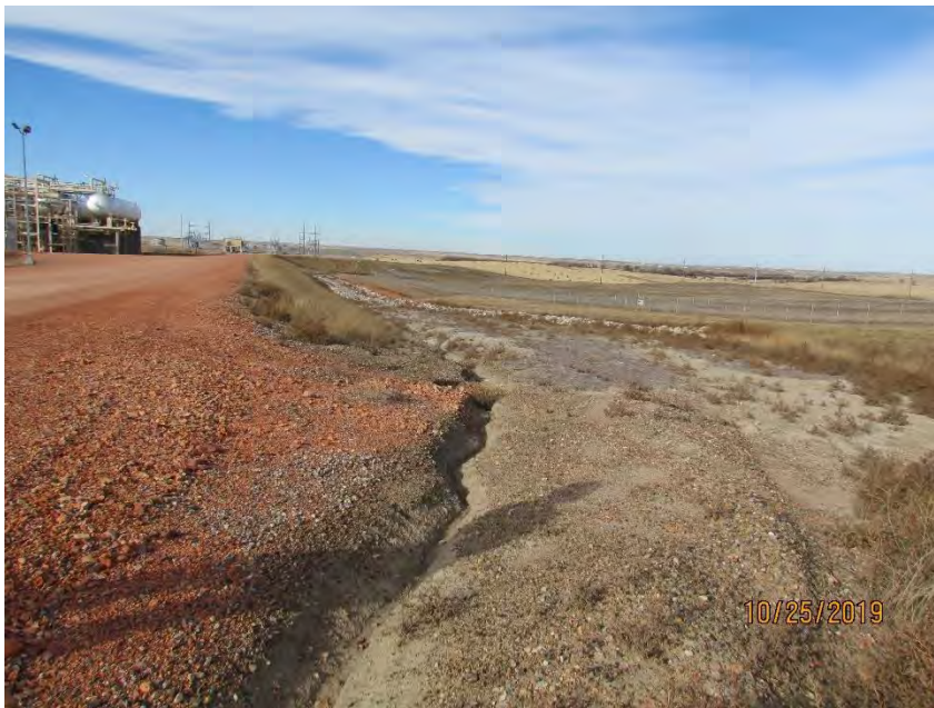
Photo 22: Gully erosion in northern extents of the facility
