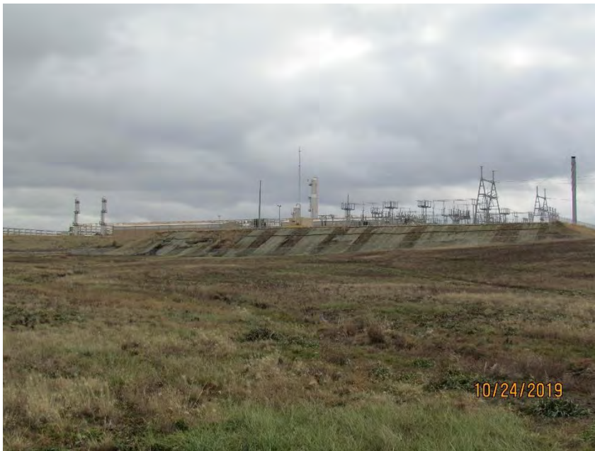
Photo 4: Facing south, view of the northwest corner of the facility. 10-24-2019
