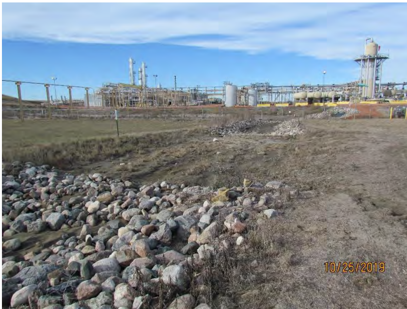
Photo 16: Stormwater drainage within the eastern extents of the facility
