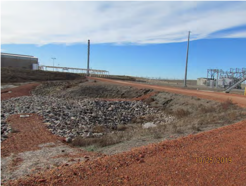
Photo 25: Facility road along northern extents of site
