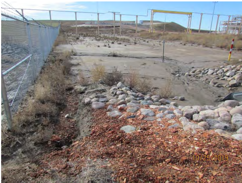
Photo 18: Facing south, view of the facility.
