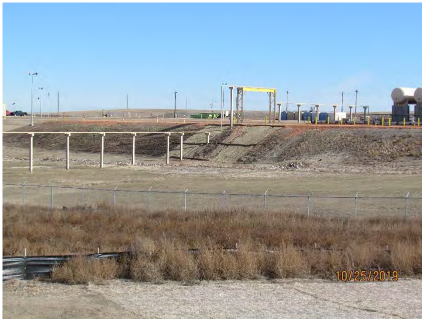
Photo 38: Facing south, view of the facility. 10-25-2019
