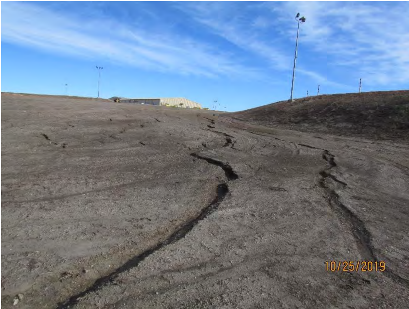
Photo 17: Stormwater flow path and gully formation along eastern portion of facility site
