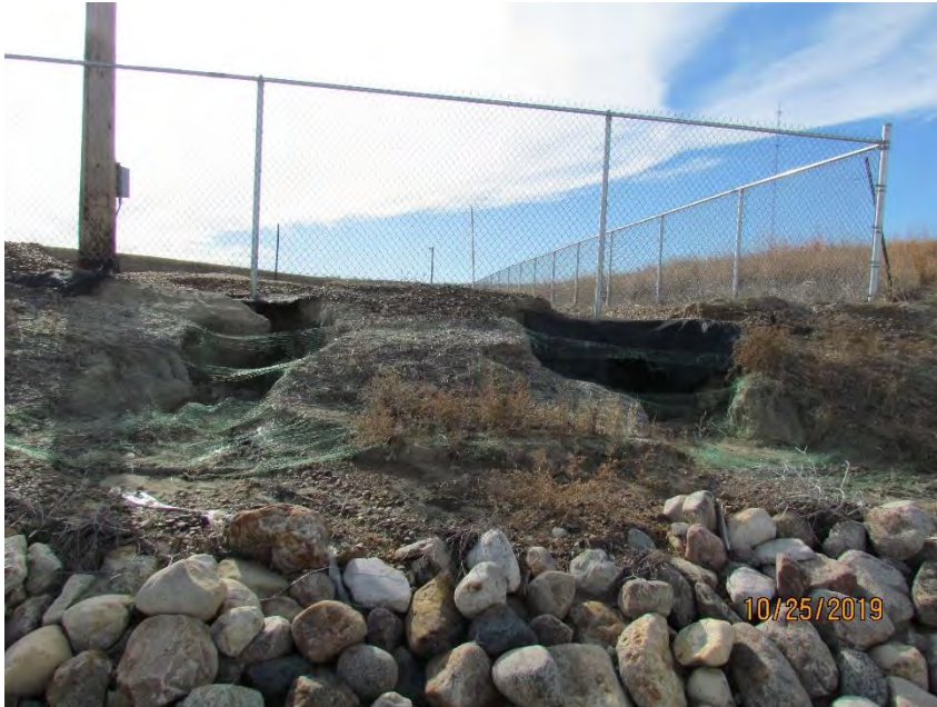
Photo 40: Stormwater conveyance path off southeastern fence line
