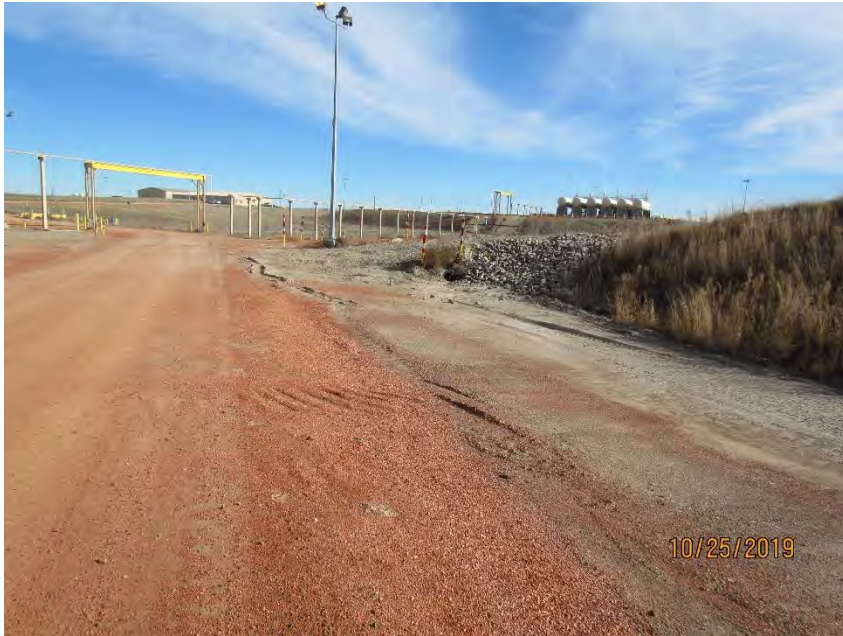
Photo 35: Facility road along southcentral portion of site 10-25-2019
