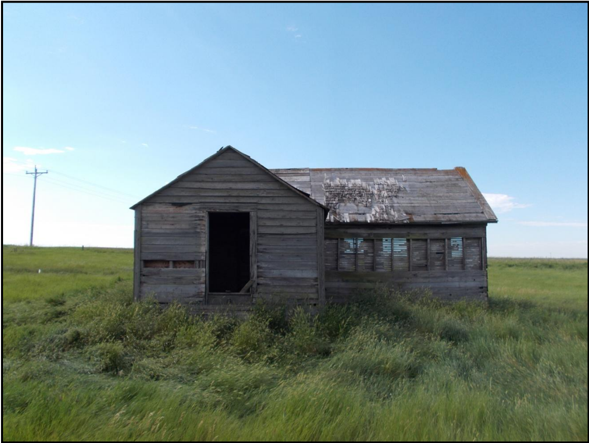
Figure 26: Overview of isolated farmhouse at 32WI1388, view to the south.
