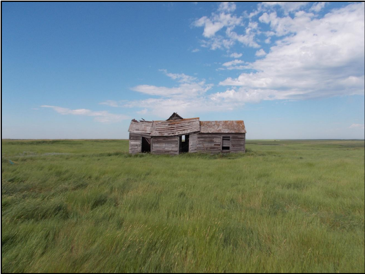
Figure 24: Overview of isolated farmhouse at 32WI1388, view to the west.
