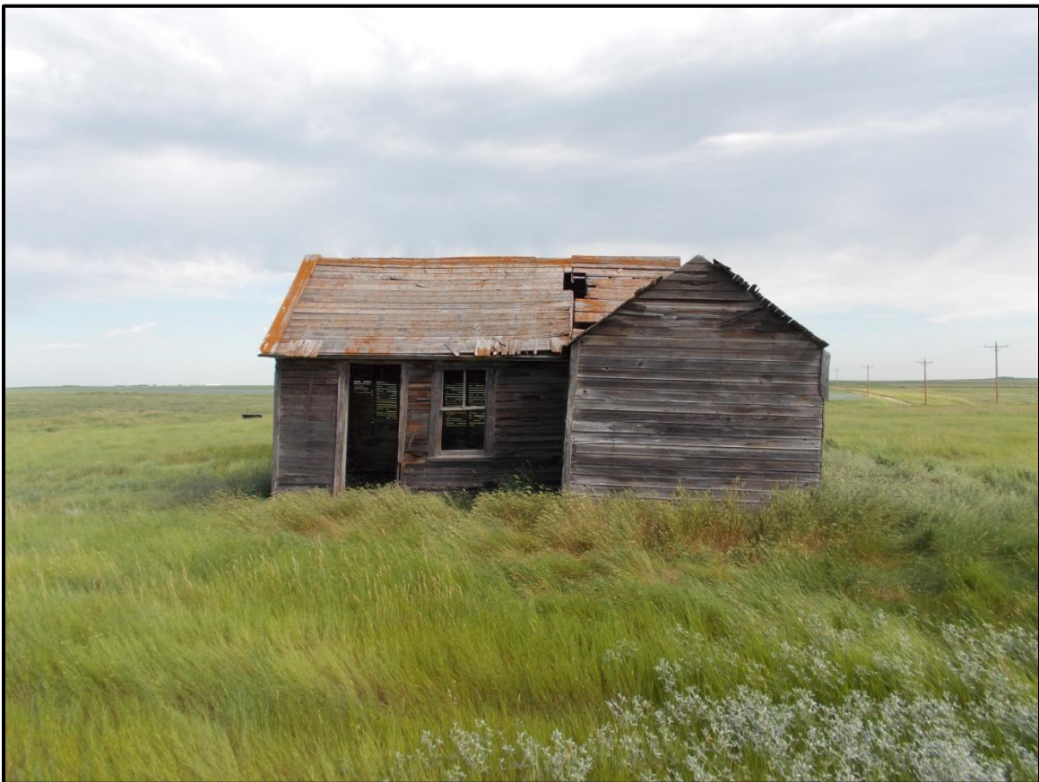
Figure 25: South elevation of the farmhouse at 32WI1388. Note crude junction of roof slopes between wings.
