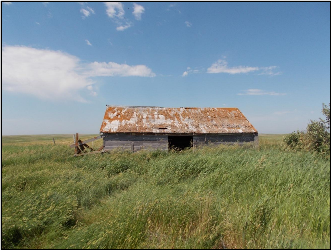
Figure 18: Overview of barn at 32DV129, view to west.
