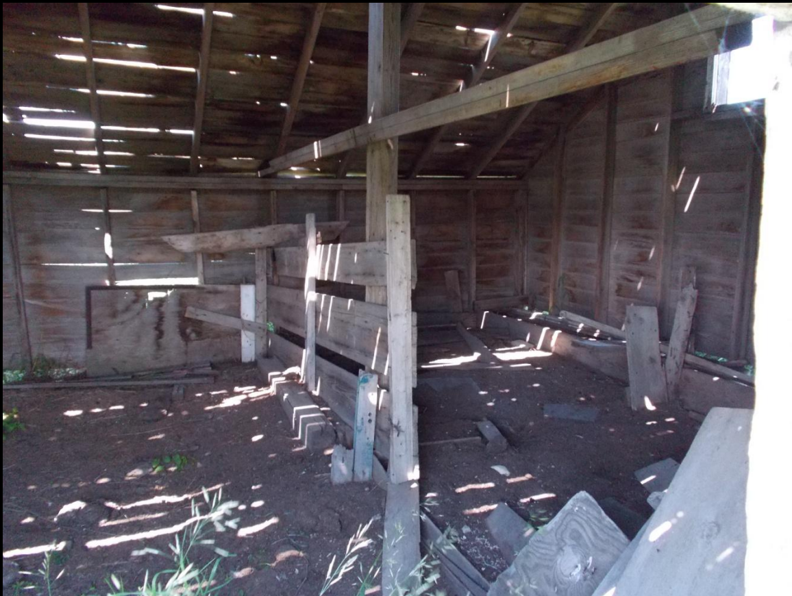
Figure 19: Overview of the inside of the barn at 32DV129.
