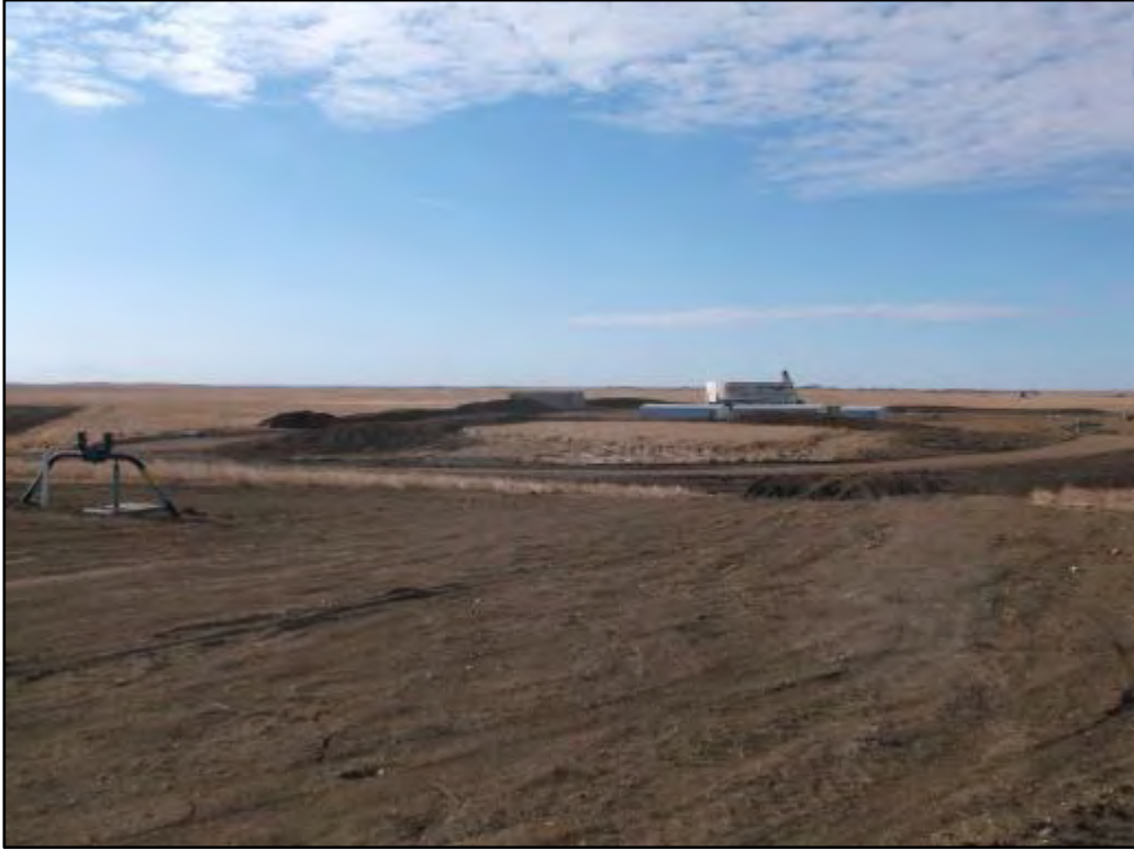
Figure C.3. Northwest corner of station, facing southeast (photo taken April 25, 2014).
