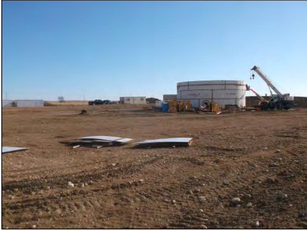
Figure C.1. Southwest corner of station, facing northeast (photo taken April 25, 2014).
