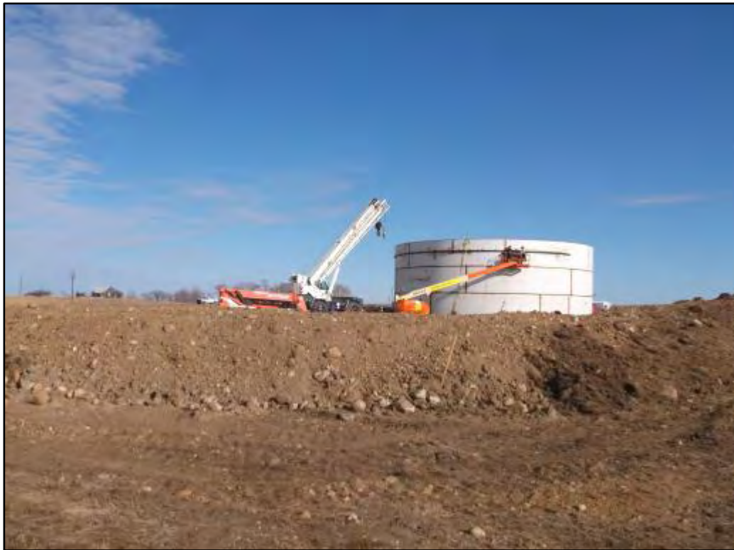
Figure C.2. Southeast corner of station, facing northwest (photo taken April 25, 2014).
