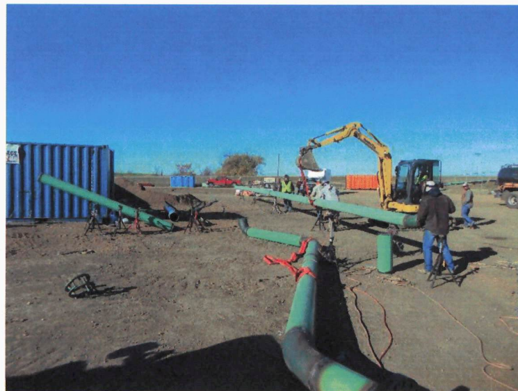
Picture 4 –Pipe welding near Fortuna, ND
