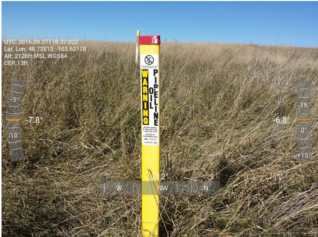
Photo 6 – Typical pipeline marker at road crossing.
