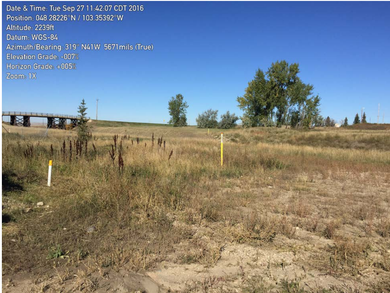
Photo 2 – Pipeline leaving CRT.
