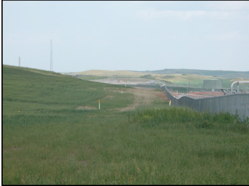
Photo 5. Direction: West. Row and pipeline corridor running east to west, three pipelines marker can be seen along the corridor.
