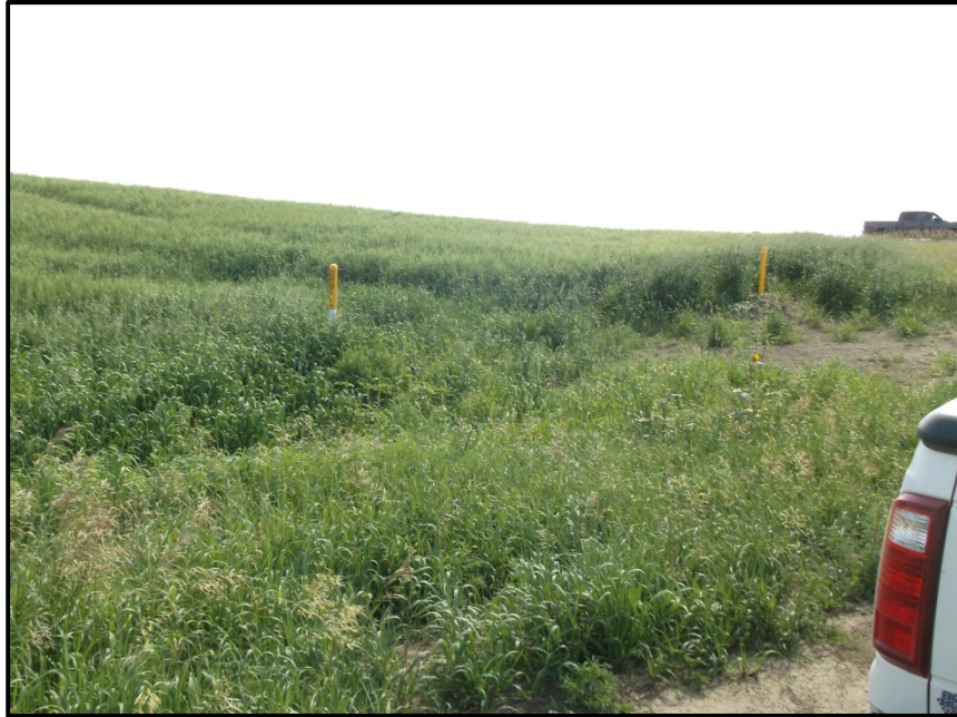
Photo 23. Direction: Southwest. Two pipeline markers show another part of the corridor that has been fully reclaimed as the pipeline bends back to west before bending again to the north.
