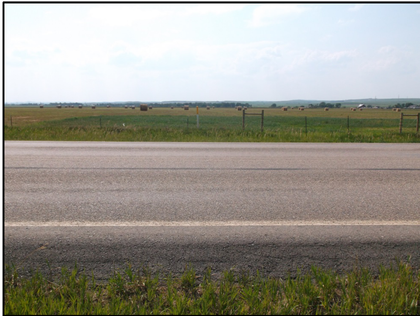
Photo 18. Direction: East. The pipeline then bends west and crosses 130 ½ Ave (the road was bored under) before it bends to the north and continues to run parallel to the road.
