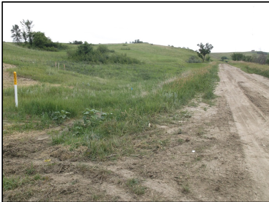
Photo 10. Direction: South. Pictured above is the pipeline corridor running East to West that still needs to be seeded and monitored to verify reclamation. A pipeline marker can be seen along the corridor. An access road that was bored under is also depicted.
