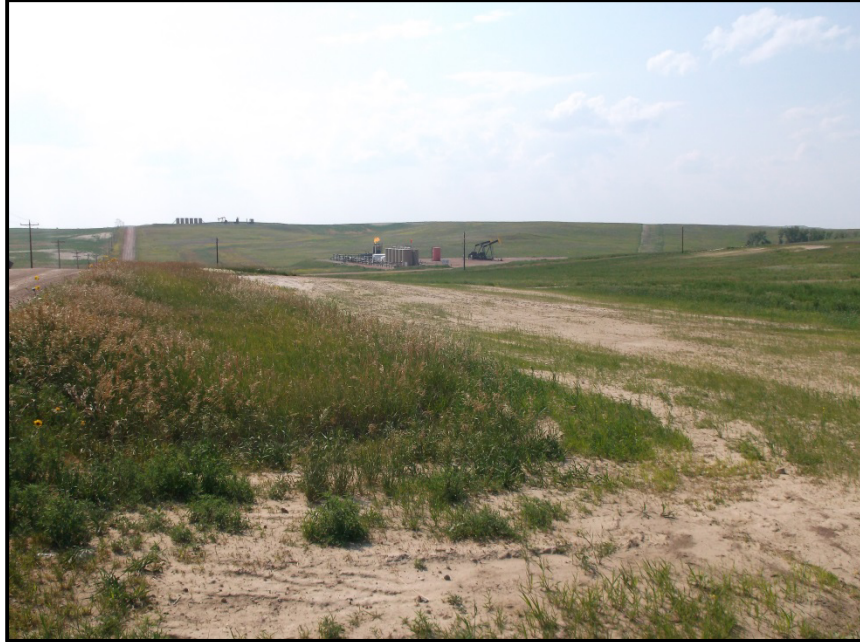
Photo 21. Direction: Northwest. Pipeline corridor as it bends away from parallel route along 20 th St and starts running through agricultural land to the northwest. This particular area needs to be continued to be monitored until seeding takes.
