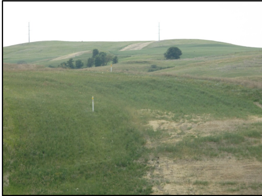
Photo 9. Direction: West. Pictured above is the pipeline corridor running East to West that still needs to be seeded and monitored to verify reclamation. Several pipeline markers can be seen along the corridor.
