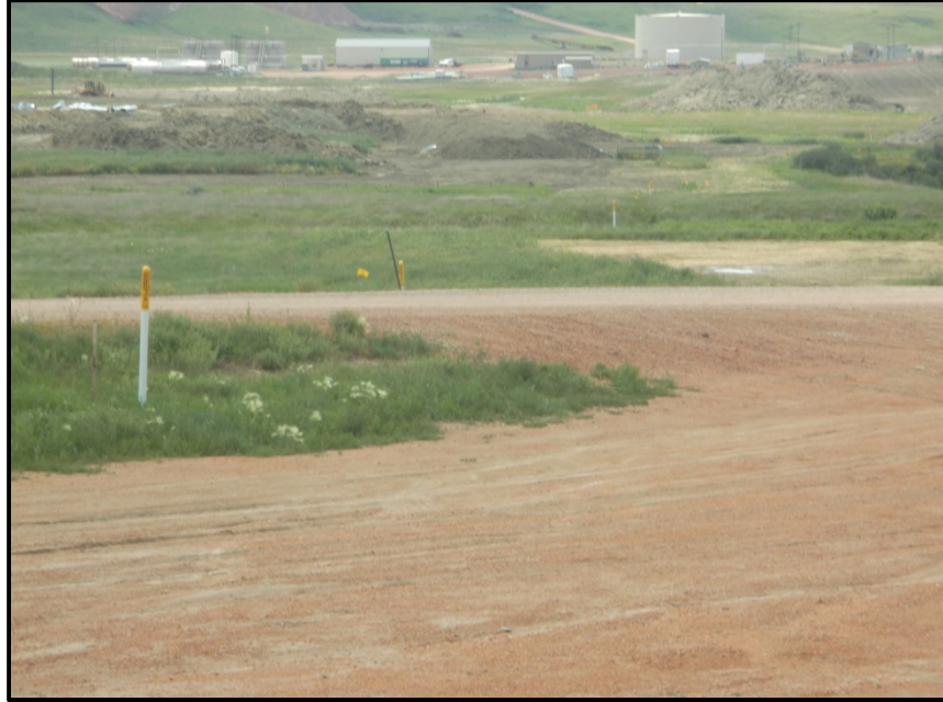
Photo 3. Direction: West. Row and pipeline corridor running east to west approaching the first crossing of an access road, four pipeline markers can be seen along the corridor.
