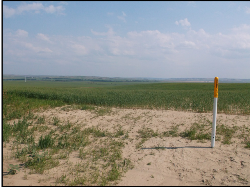
Photo 19. Direction: East. This marker signifies a bend to the west where the pipeline will run parallel to 20 th St. This area of rural land has been restored to preconstruction conditions.
