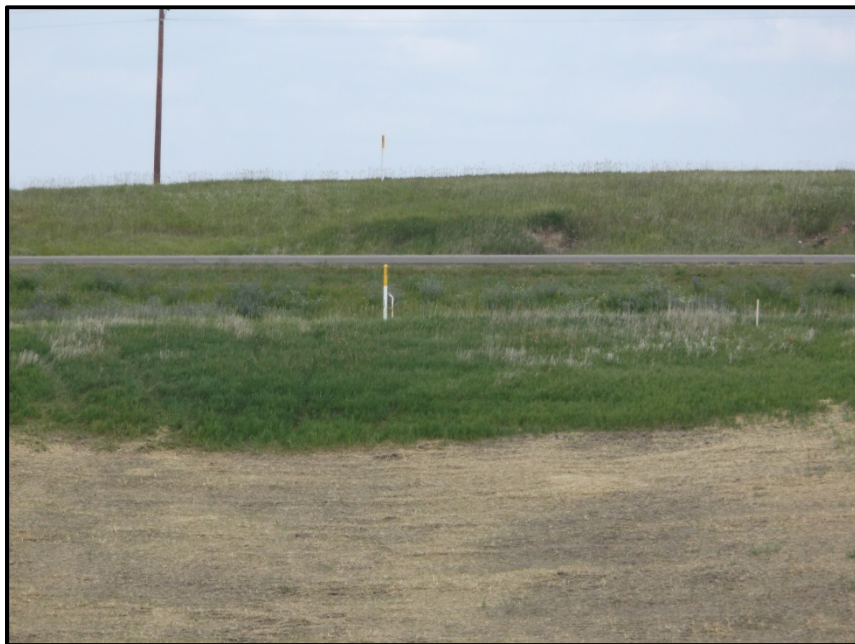
Photo 6. Direction: West. Row and pipeline corridor running east to west approaching the crossing of Highway 85, two pipeline markers can be seen along the corridor. Areas of the corridor that need to be seeded are shown as well.
