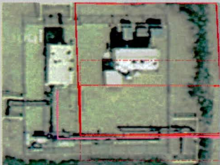
Hawthorn Pump Station
