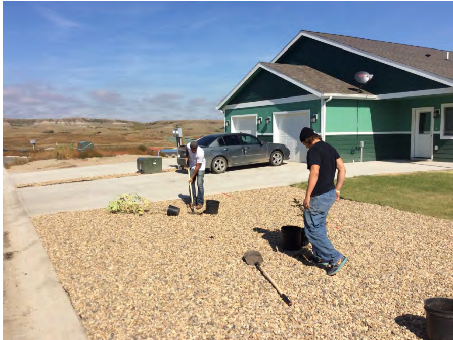
Photo B.11-1 TC Nursery employees in the process of preparing planting locations and planting trees.
