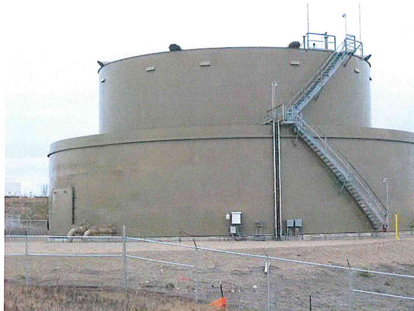
Photo 16 – View of Stanley tank facilities.
