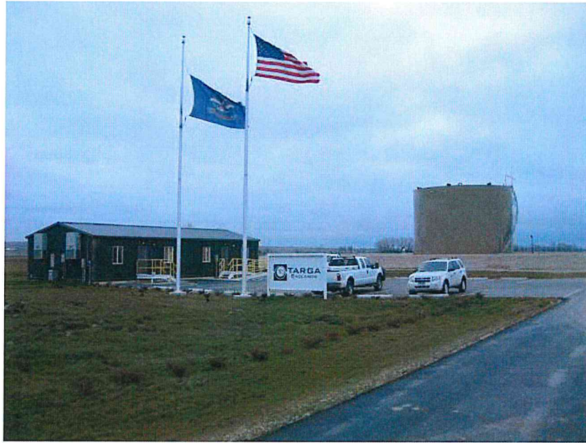
Photo 1 – View of Targa New Town tank facilities.
