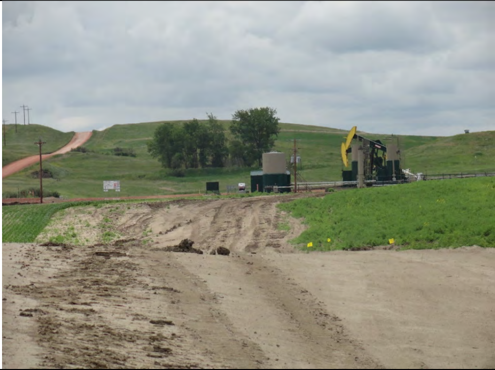
Photo Log Point 13: Pipeline route looking west (trees at Photo Log Point 12)
