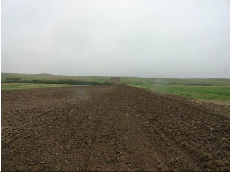
Photo Log Point 3: Pipeline route looking south
