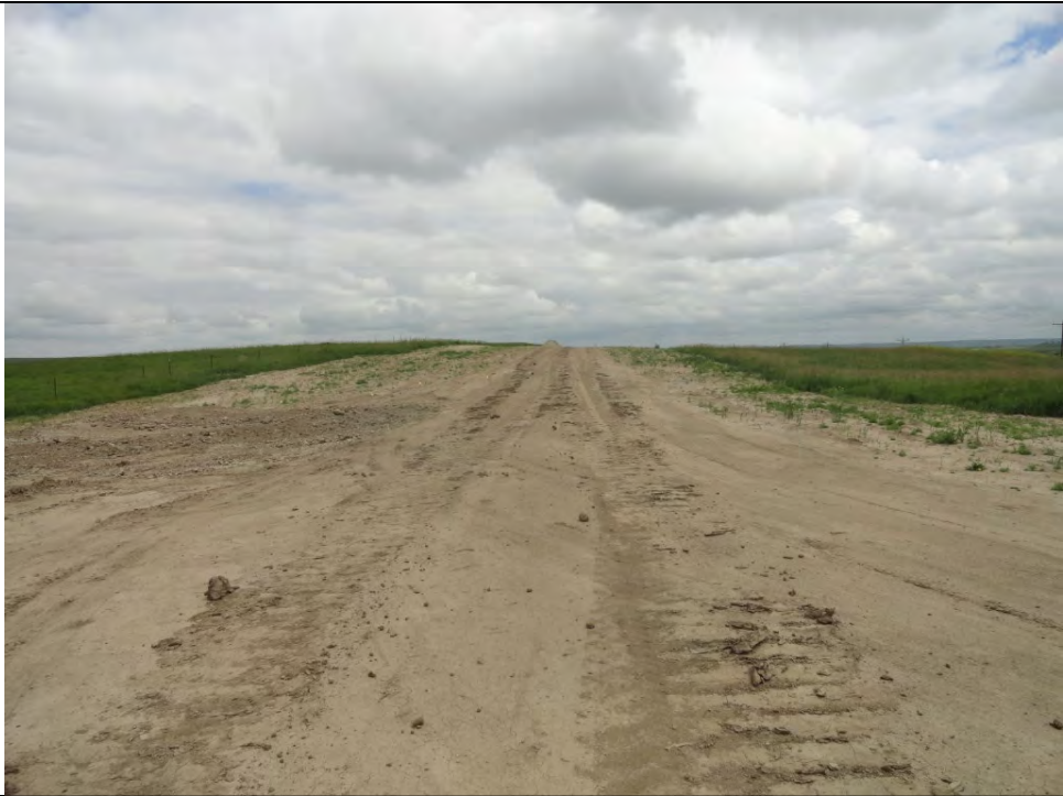
Photo Log Point 13: Pipeline route looking east
