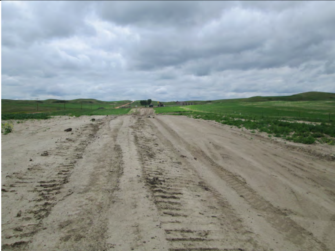
Photo Point 11 – Facing west, this section of pipeline has been restored
