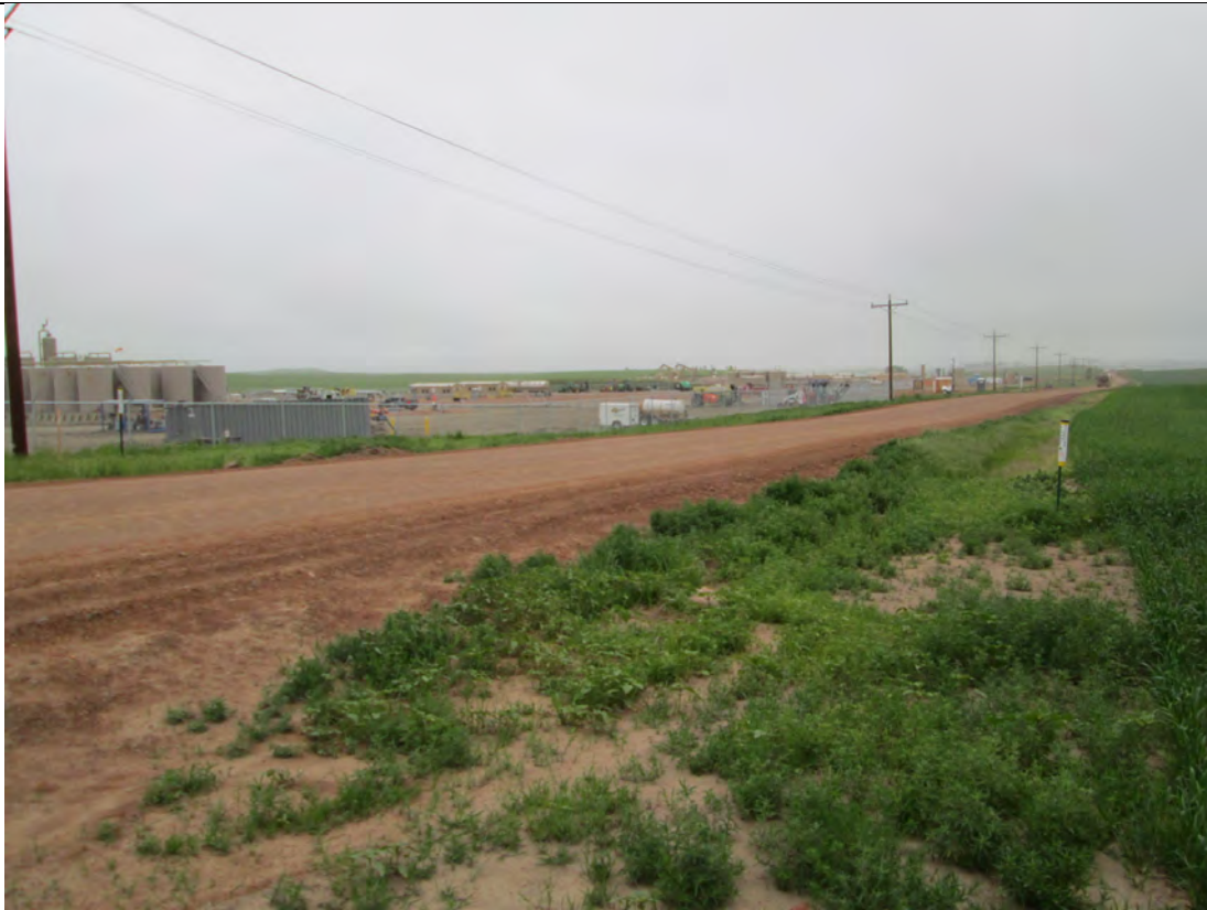
Photo Point 1 – Looking northeast at main facility
