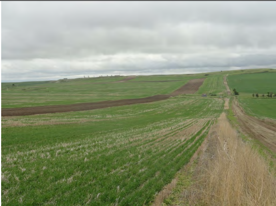
Photo Log Point 7: Pipeline route looking north
