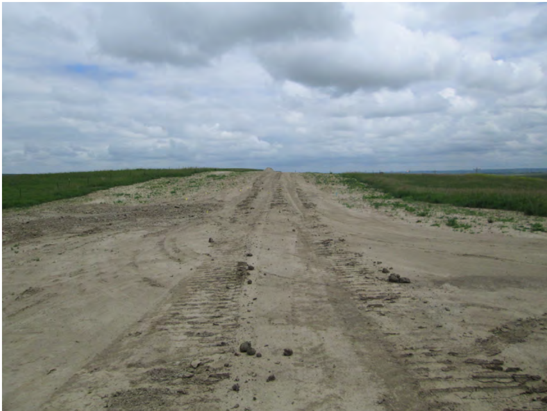
Photo Point 11 – Facing east, this section of pipeline has been restored
