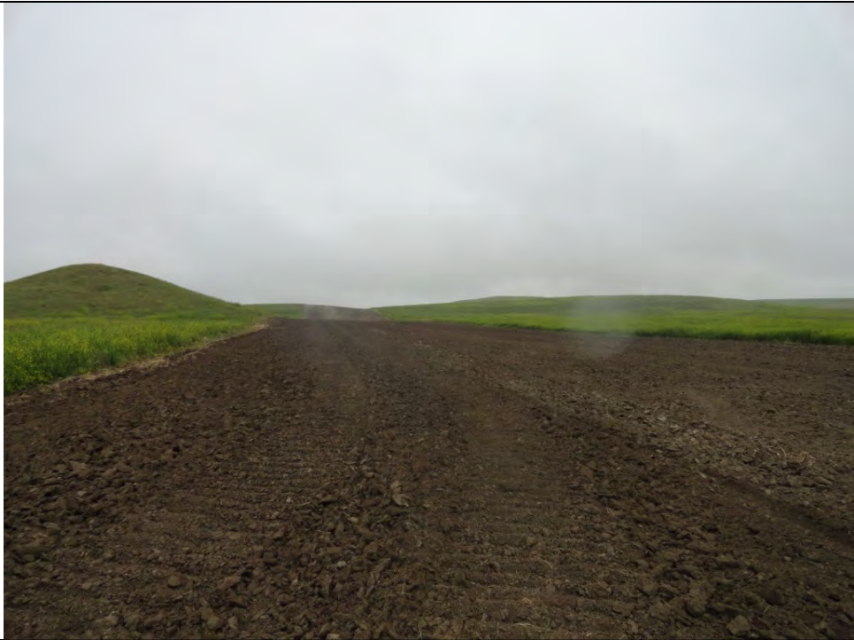
Photo Log Point 3: Pipeline route looking north
