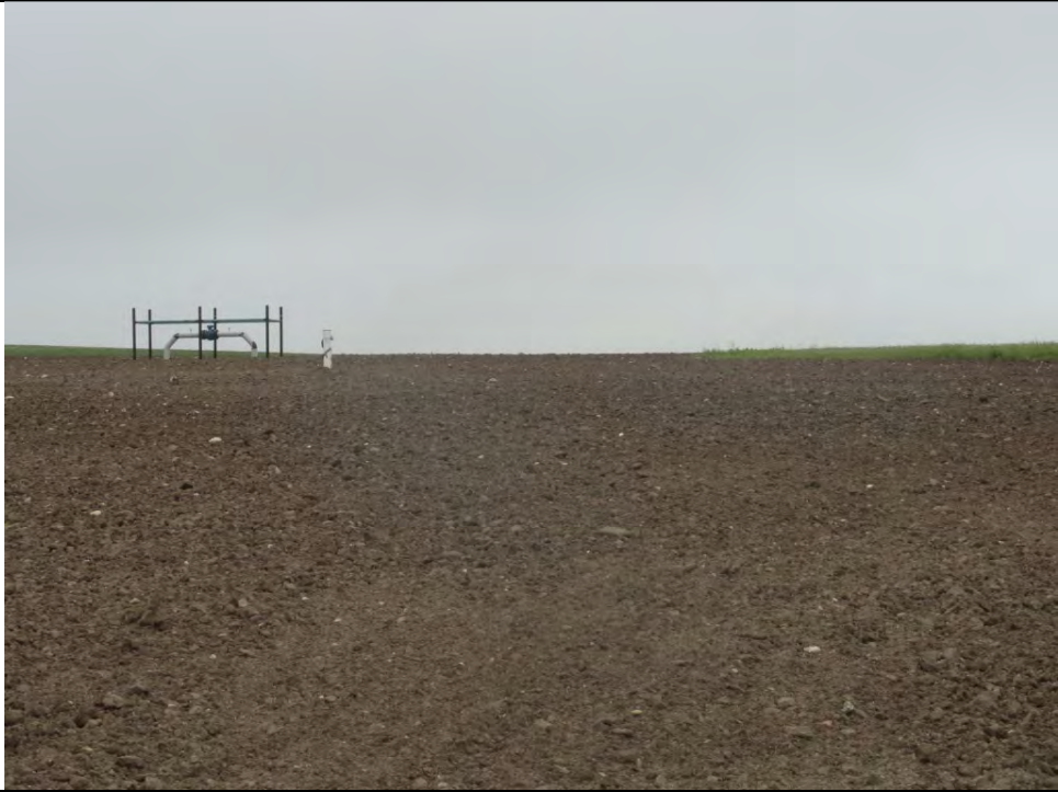
Photo Log Point 1: Above ground pipeline feature south of Hey Butte facility
