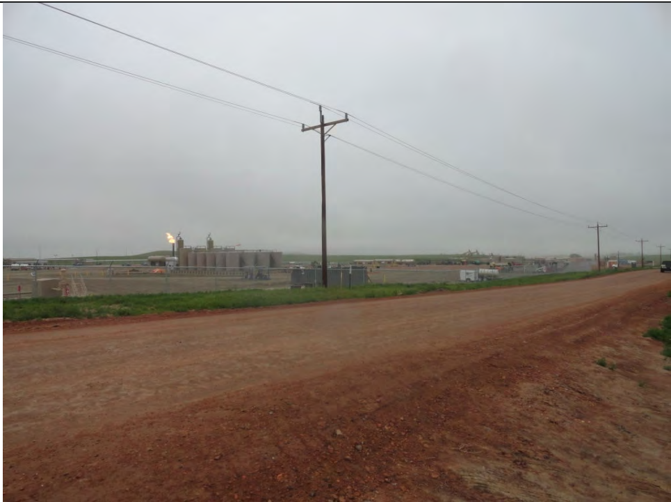
Photo Log Point 1: Hey Butte Facility (2)
