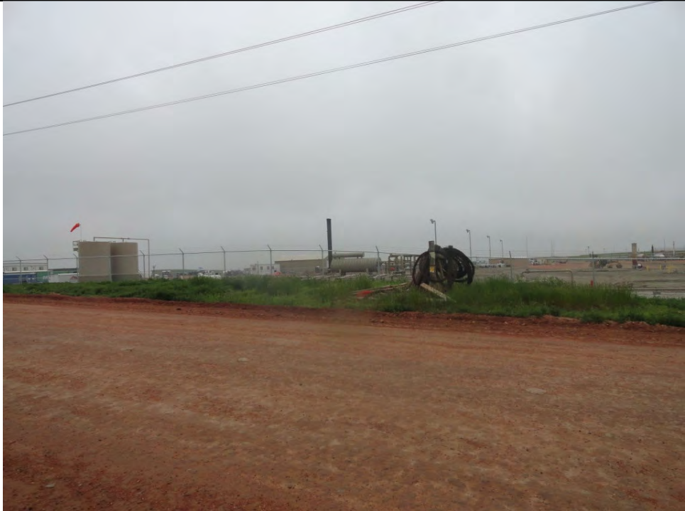
Photo Log Point 1: Hey Butte Facility (1)
