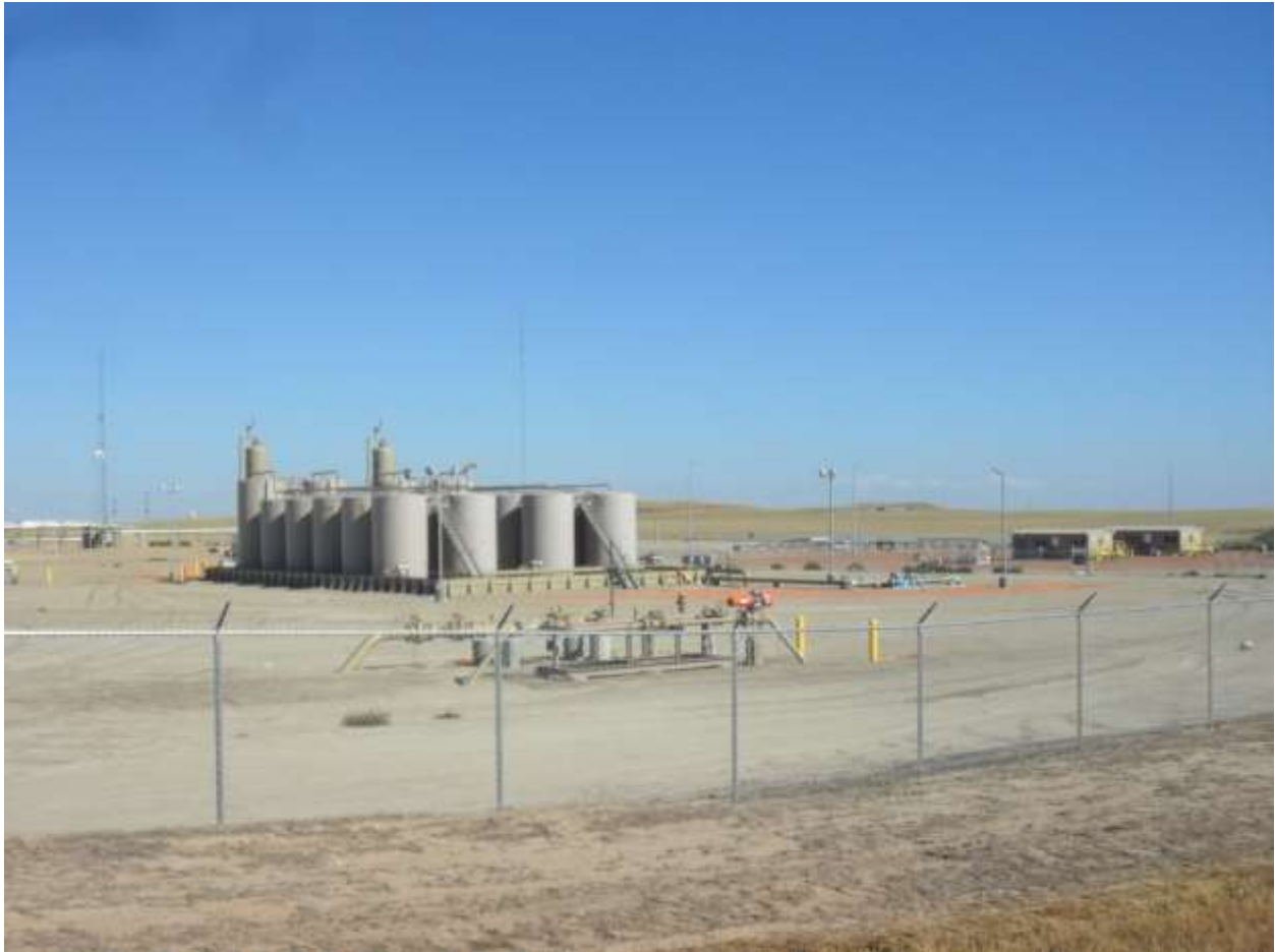
Photo 2 – Hay Butte Plant, pipeline start.
