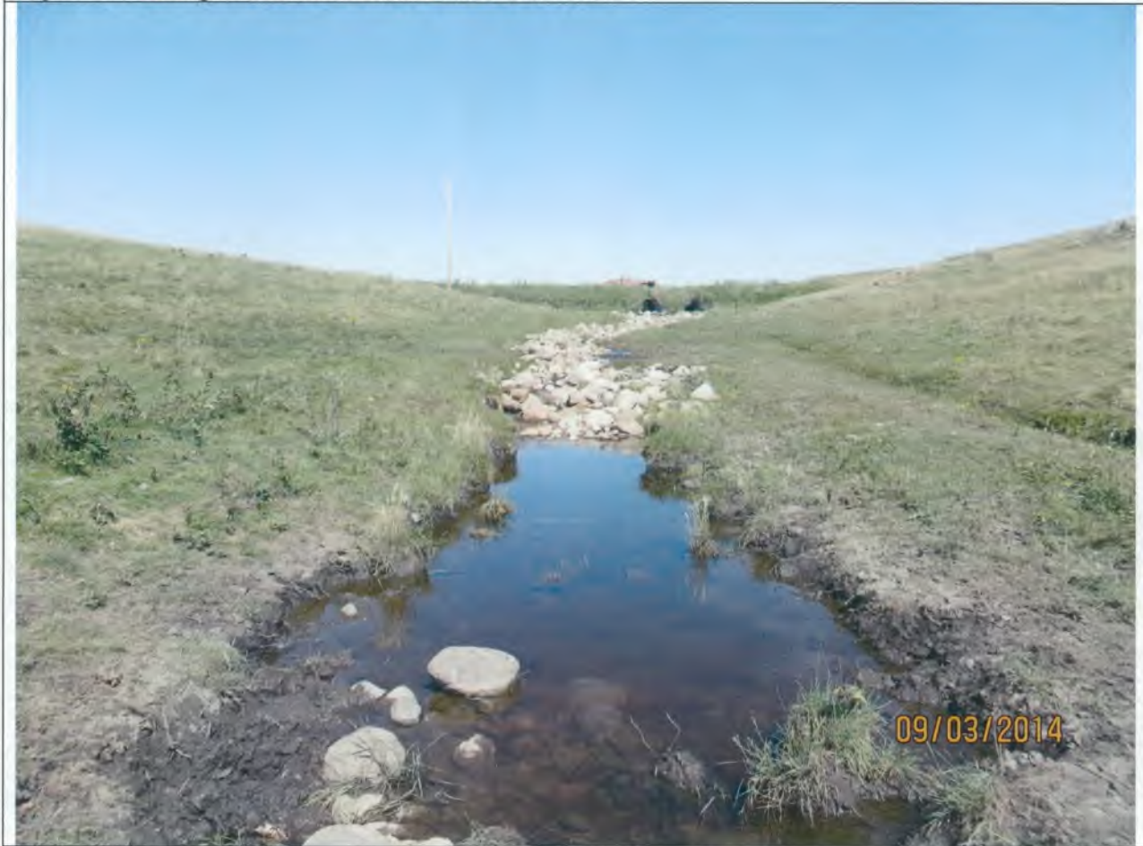
Figure 5: Drainage in Section 7 where runoff is diverted
