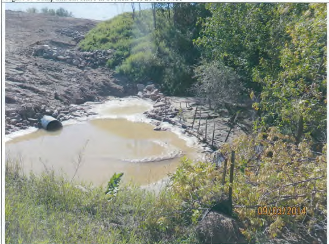
Figure 3: Sump and silt fence in Section 5 of BNCR-9401
