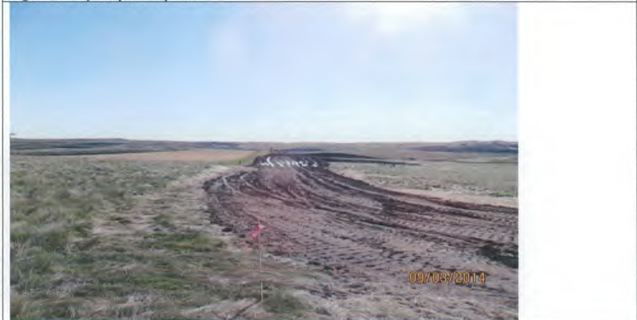
Figure 1: Topsoil pile off permit
