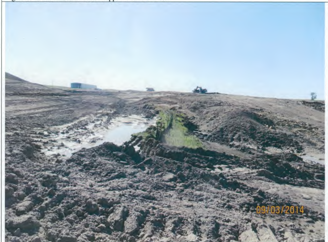
Figure 4: Soil that needs to be stripped from BMP site
