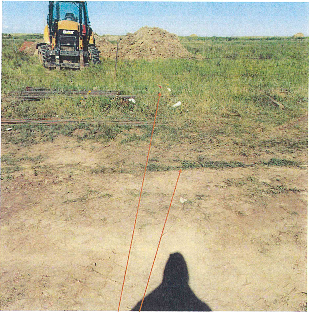
Looking West across construction area
