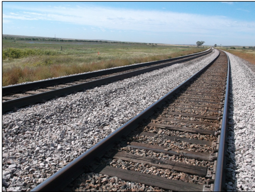
Figure 2. 32WI481 site overview, facing south.
