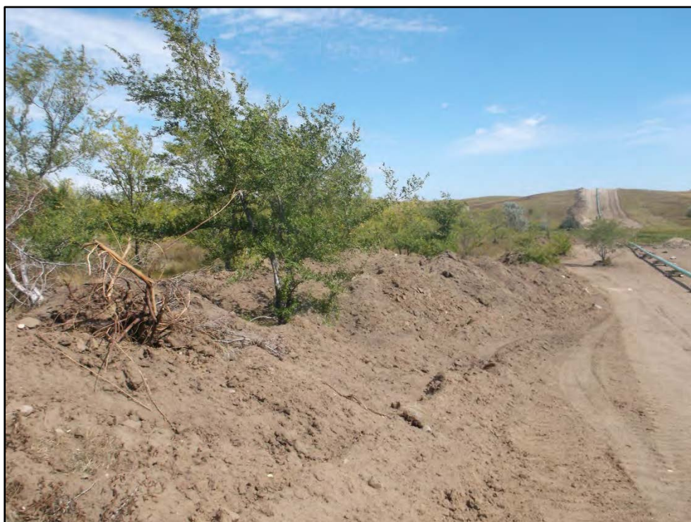
Figure B.24. Overview of BWV5, facing northwest.
