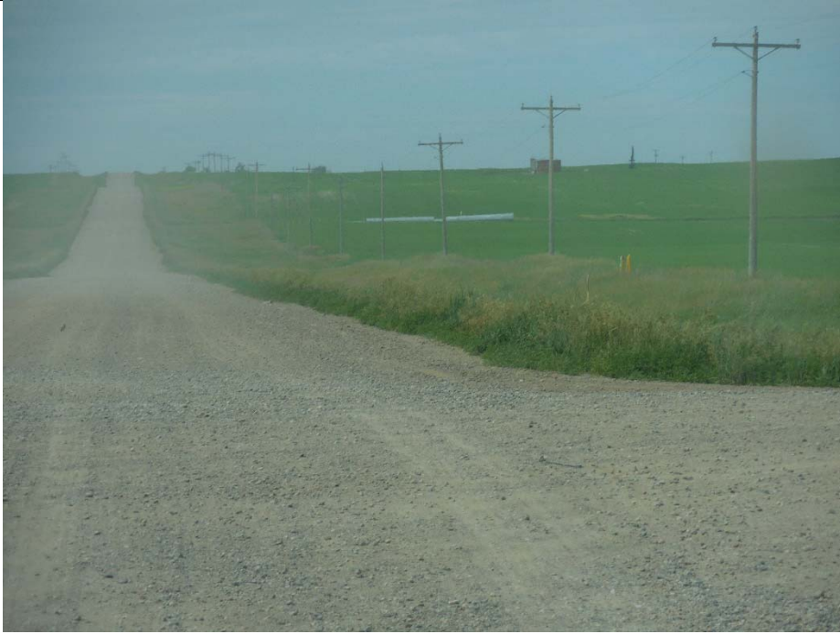
Photo 8: Pipeline corridor at intersection of County Highway 11 and Co and County Road 8, facing west. Corridor is on the north (right) side of the road.
