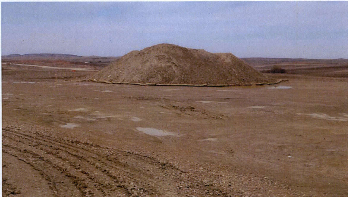
Photo 3. Subsoil pile on level surface, protected by waddles.
