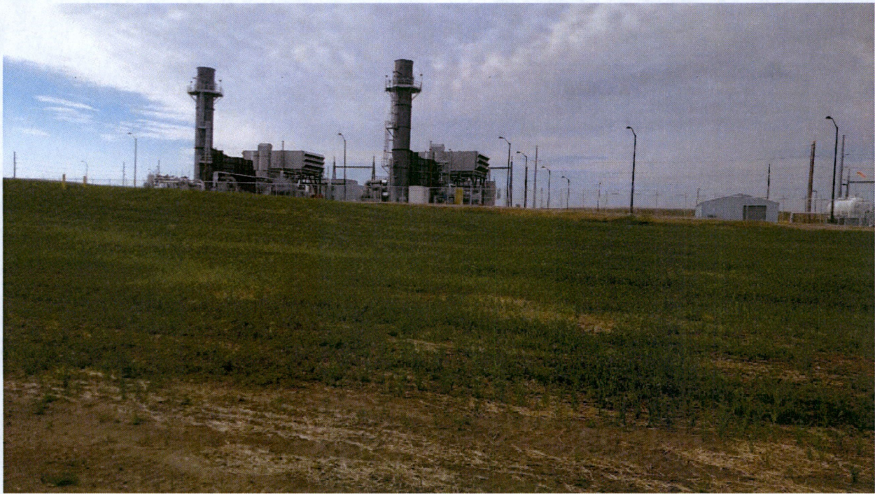
Photo 1. Reclaimed (in process) portion of Project Site.
