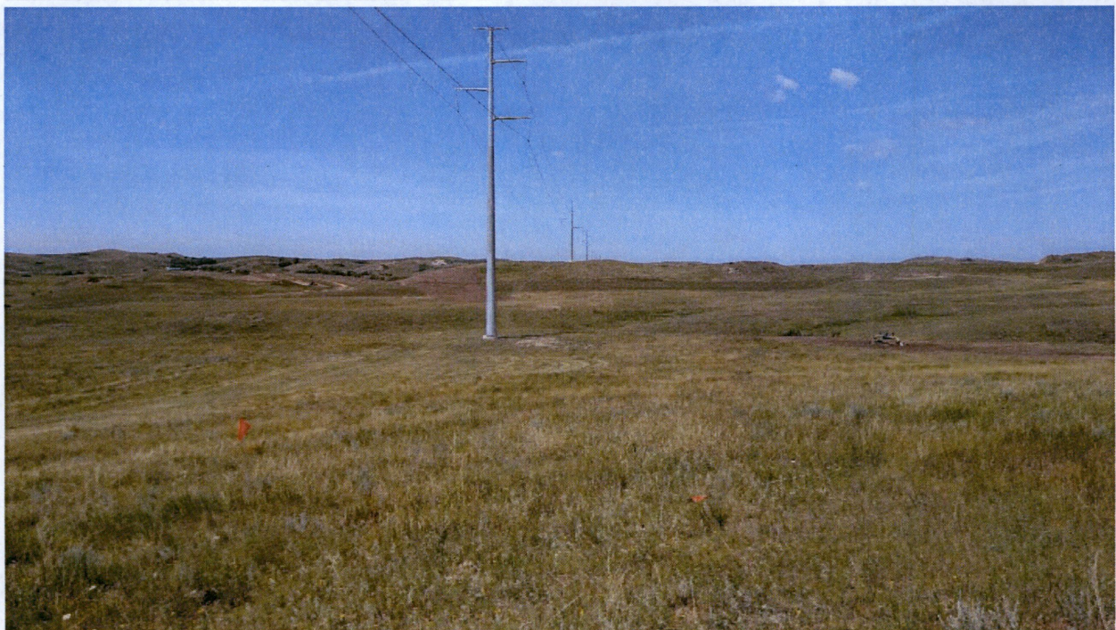
Photo 5. Strung towers spanning recent pipeline project.
