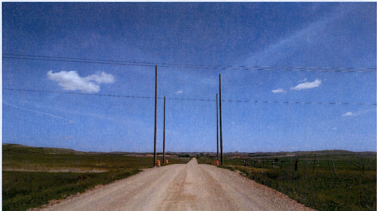
Photo 6. Supports for spanning wire across road.
