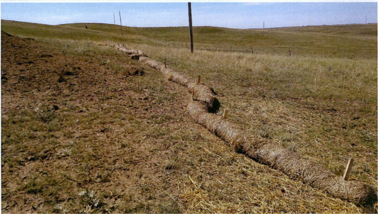
Photo 3. Properly-installed wattle on downhill slope of crane pad.
