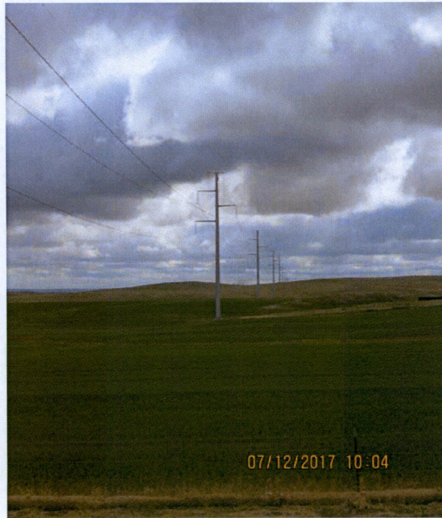
Photo 5: Looking east at structure 24, no concerns identified.
