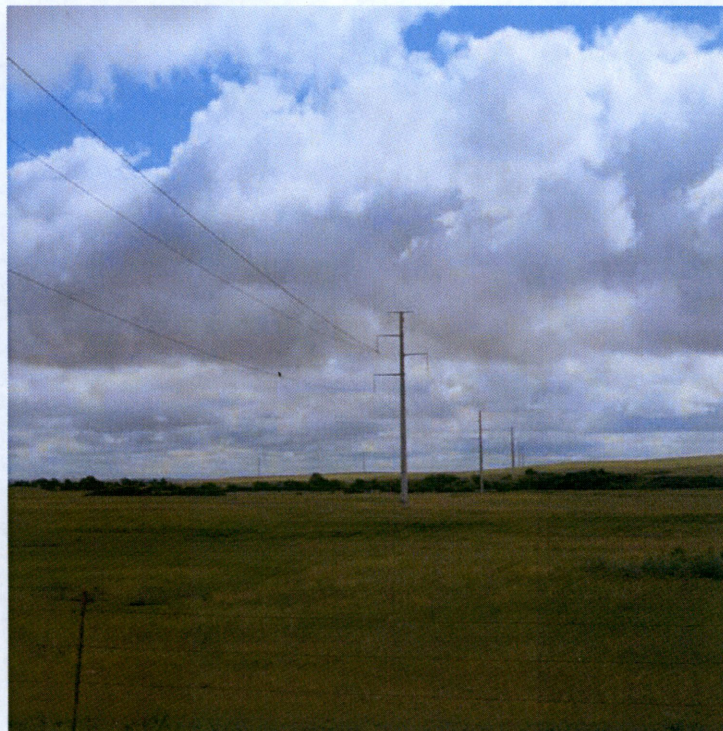
Photo 7: Looking east at structure 48, no concerns identified.
