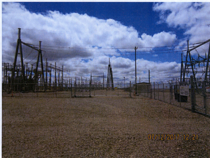
Photo 12: Kummer Station, no concerns identified.
