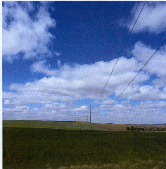
Photo 11: Looking west at structure 154.
