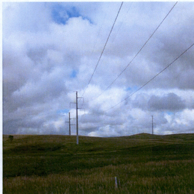
Photo 6: Looking southwest at structure 36, no concerns identified.
