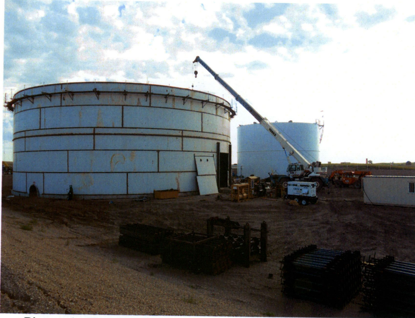
Picture 1 - New 50,000 barrel breakout tank under construction
