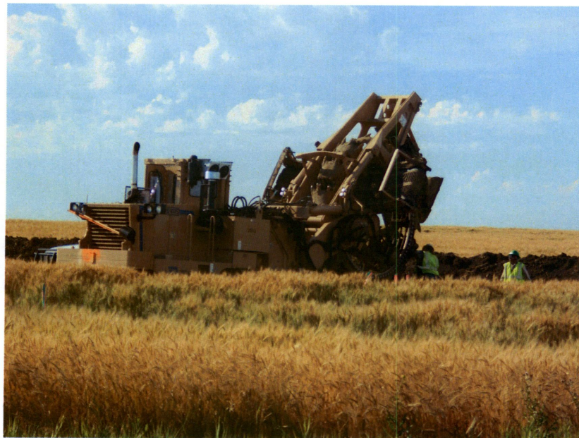
Picture 8 - Pipe Trenching Machine
