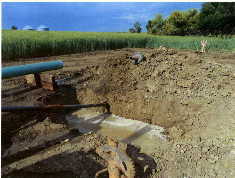
Picture 10 - Pilot Hole being bored
