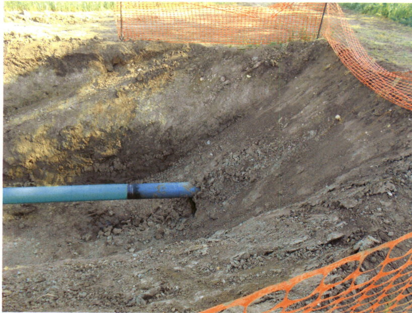
Picture 7 - Intersection of Bore Pipe and Standard Epoxy Covered Pipe
