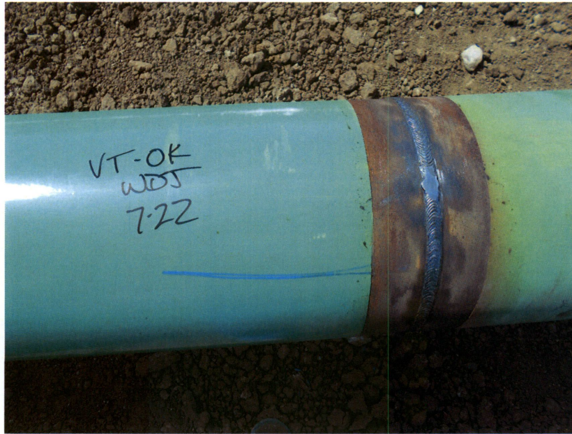
Picture 13 - Typical Pipe Weld and Inspection Marking
