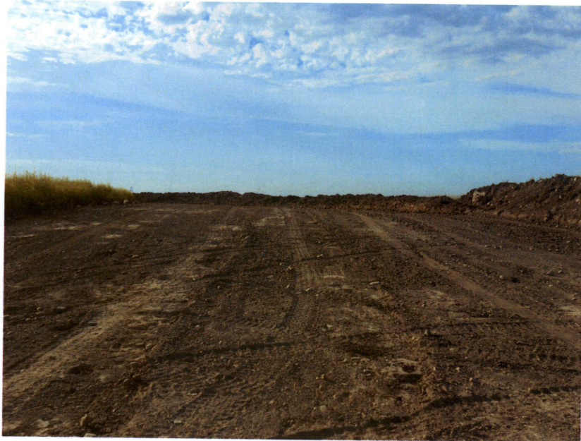
Picture 5 - West End – Trench Backfill
