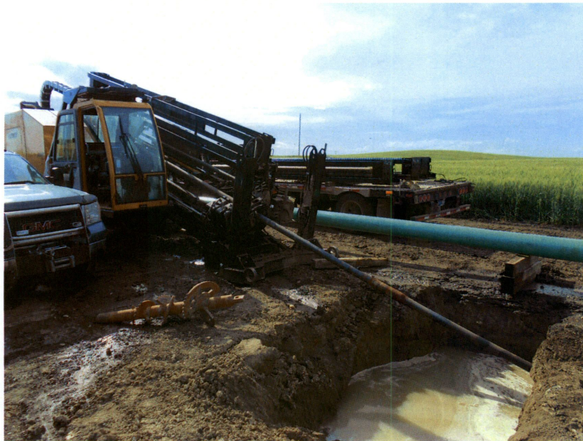
Picture 9 - Soil Hole Boring Machine
