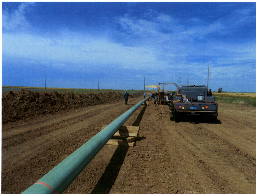
Picture 12 - East End – Pipeline Welding Crew
