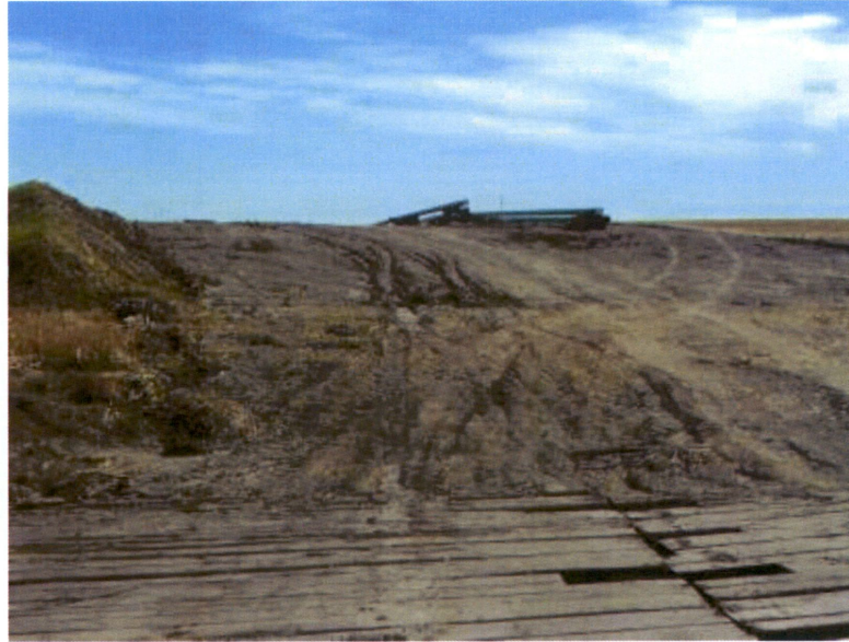
Picture 9 - Typical matting set at critical areas
