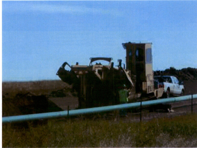
Picture 7 - Piping trencher in operation
