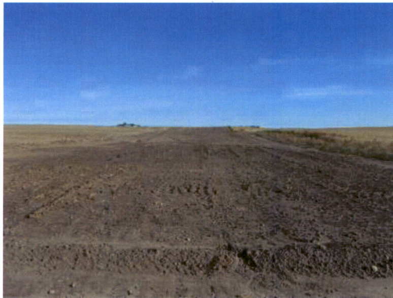
Picture 4 - Typical area where backfill and grading have taken place
