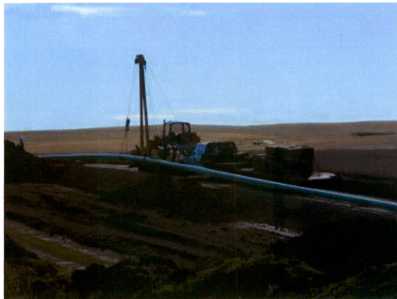
Picture 8 - Pipe being placed in trench
