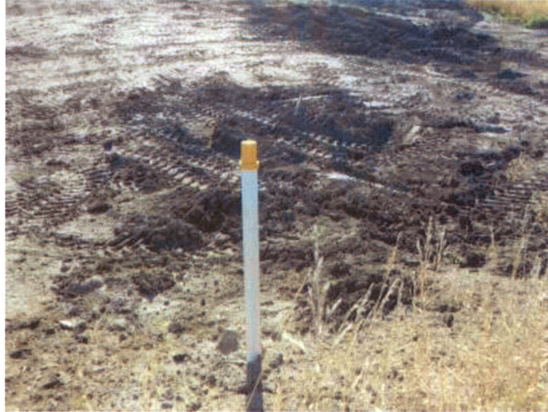
Picture 5 - Typical piping cathodic protection point
