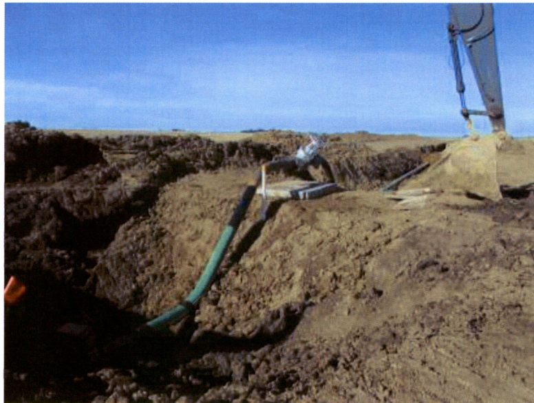
Picture 6 - Block valve station #3 being installed
