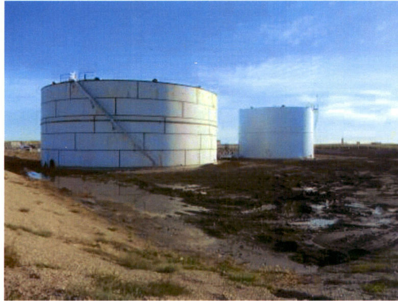
Picture 1 - New 55,000 barrel storage tank nearly completely constructed
