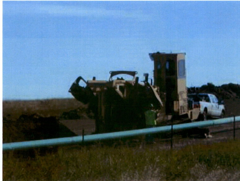
Picture 7 - Piping trencher in operation
