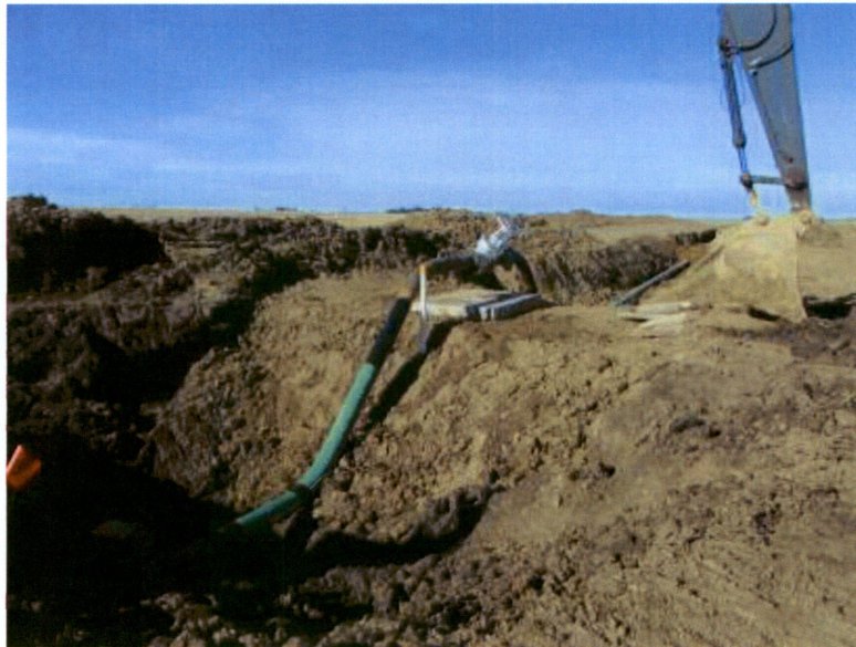
Picture 6 - Block valve station #3 being installed
