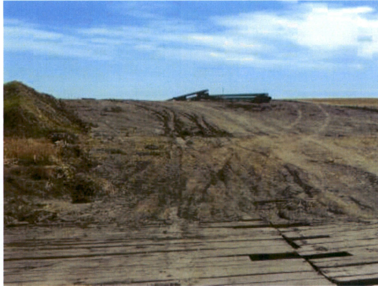
Picture 9 - Typical matting set at critical areas
