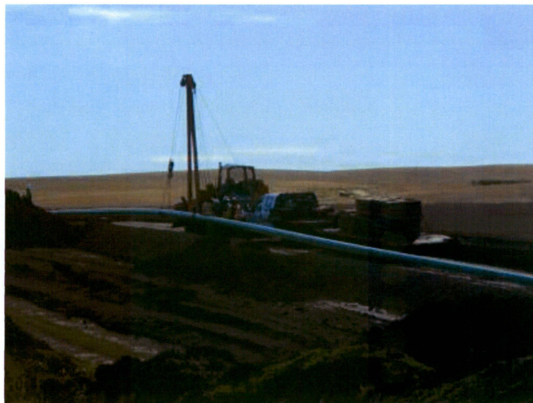
Picture 8 - Pipe being placed in trench
