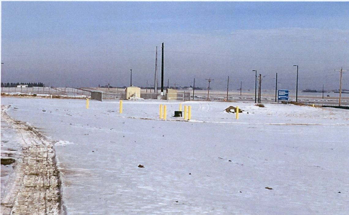
Photo 12 – View of natural gas line route
