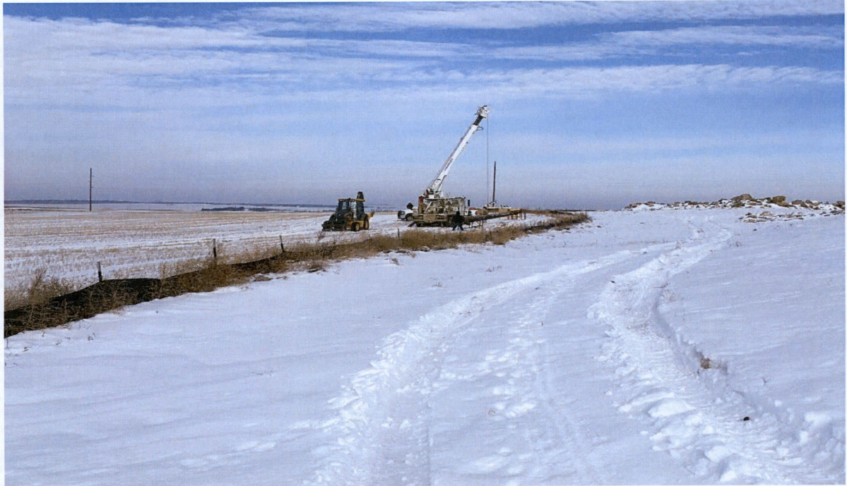
Photo 13 – View of electric transmission line construction
