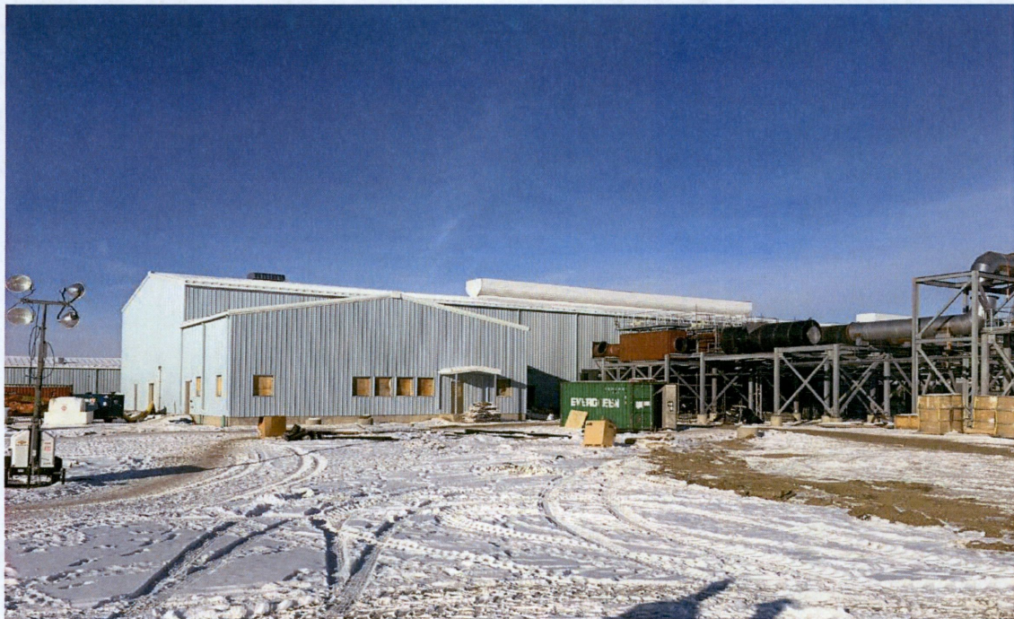
Photo 2 – View of Pioneer Generation Station Phase III facilities
