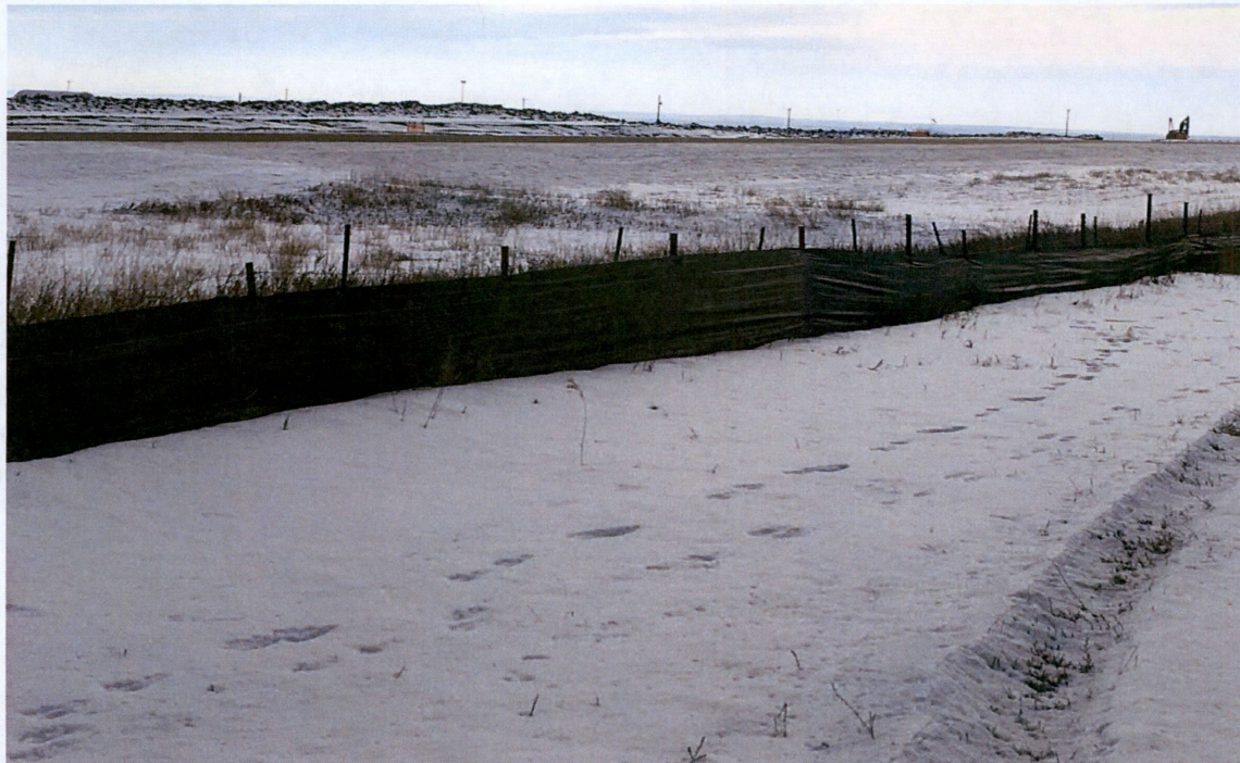
Photo 8 – View of silt fence along the perimeter of the site
