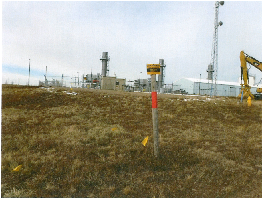
Photo 9 – View of restored gas pipeline corridor.
