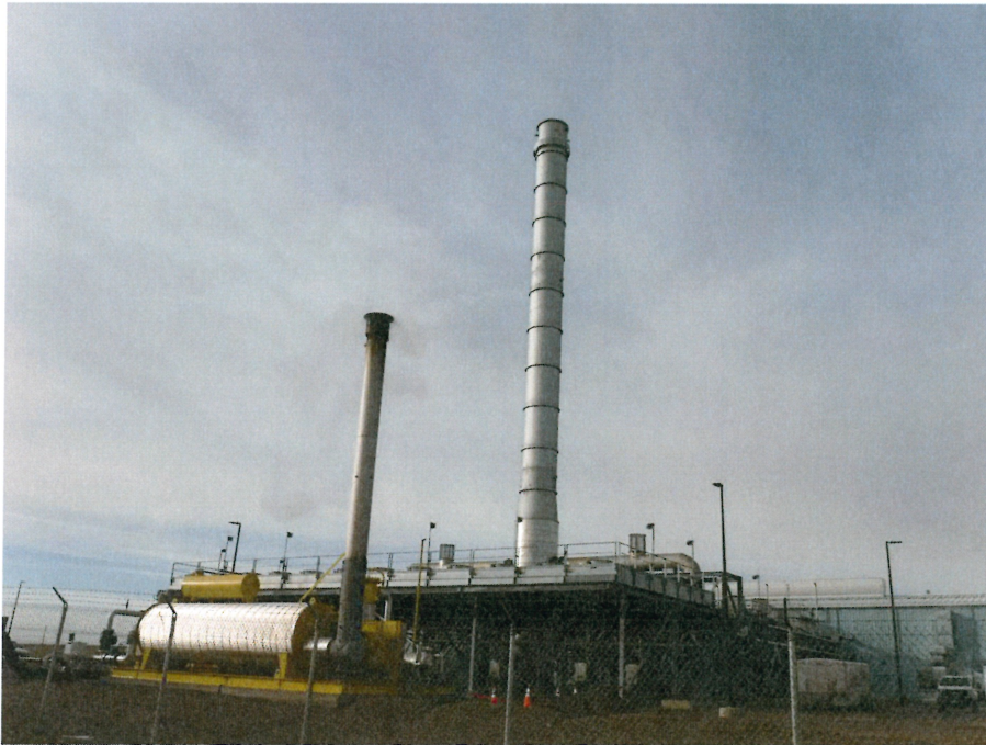
Photo 2 – View of Pioneer Generation Station Phase III facilities.
