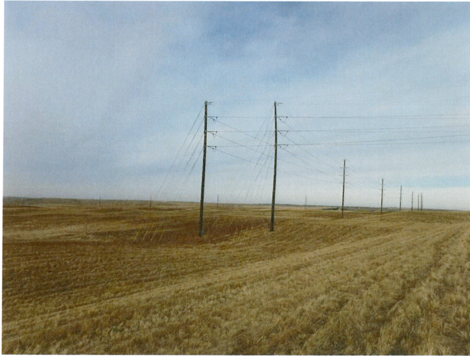
Photo 7 – View of restored power line corridor.
