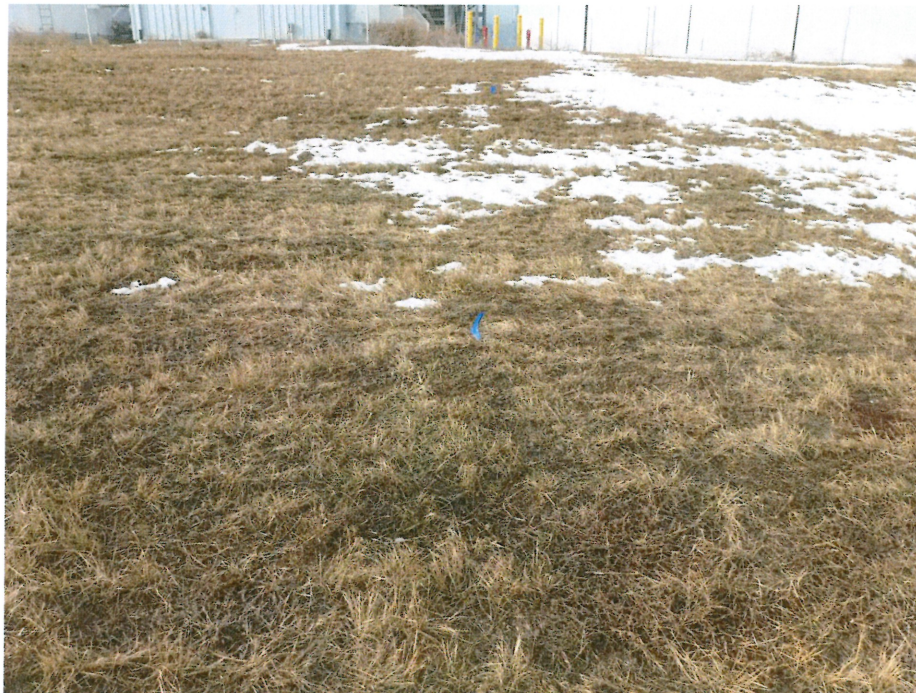
Photo 10 – View of restored water line corridor.
