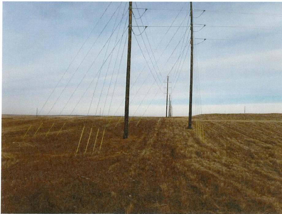
Photo 8 – View of restored power line corridor.
