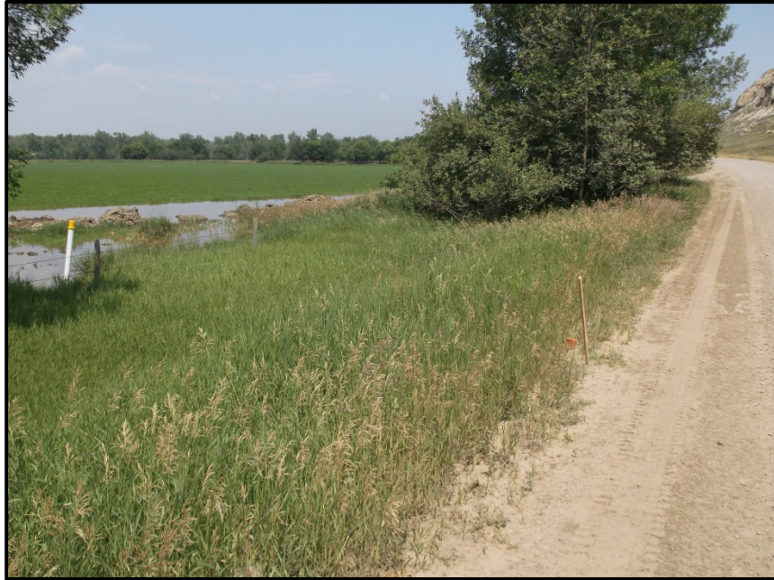
Photo 11. Direction: North. After the bore underneath the river the pipeline continues to the east.
