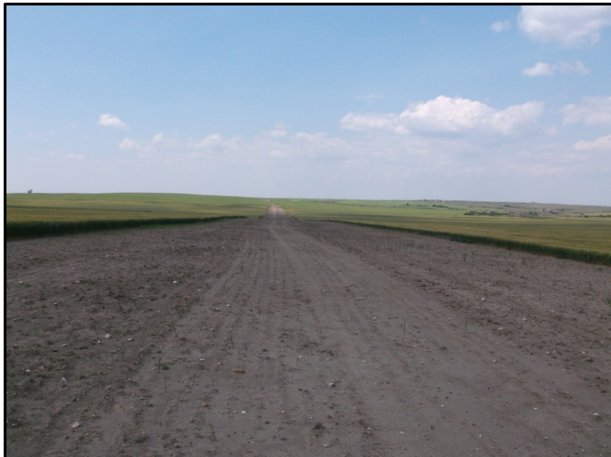
Photo 32. Direction: East. This portion of the corridor was recently seeded and needs to be monitored until fully reclaimed. It was apparent that the route corridor widths described in the application were used throughout the project as depicted in the picture above.
