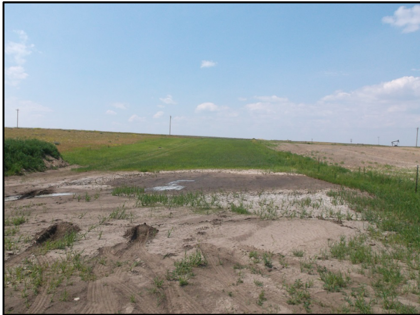
Photo 34. Direction: East. The pipeline corridor continues to run east to west through farmlands. The area has been seeded and will be returned to preconstruction conditions.
