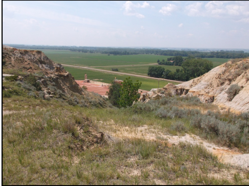
Photo 13. Direction: West. This is the approximate exit point of the bore through the hill. The pipeline then continues to the east following the existing ground contours.
