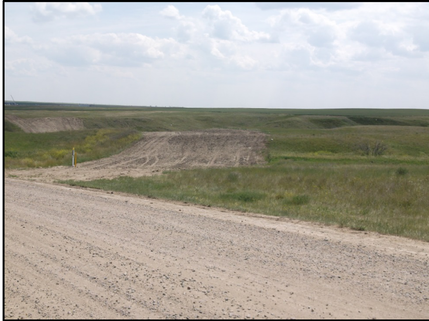
Photo 23. Direction: Southeast. The pipeline crosses 36 th St NW and runs north of the road for a short while before crossing again and continuing parallel and south of the road. This portion of the corridor still needs to be seeded and monitored until fully reclaimed.
