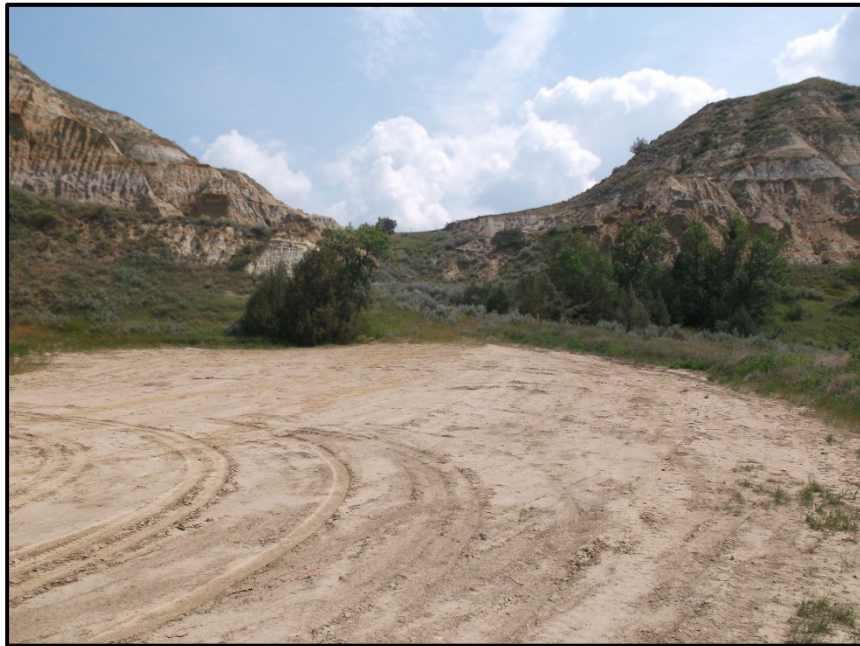
Photo 12. Direction: East. The pipeline continues to the east and a bore was completed through the hill pictured above.
