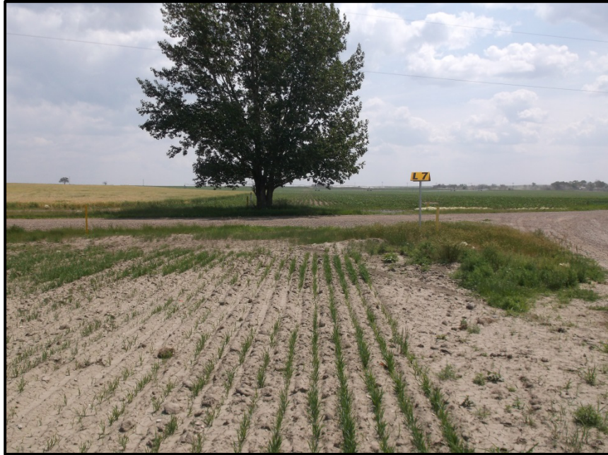
Photo 19. Direction: East. This section of the pipeline ROW runs east and west before bending to the southeast and has recently been seeded as depicted above. A follow up by the PSC with Kinder Morgan is needed to ensure full reclamation.
