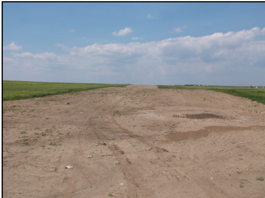
Photo 30. Direction: East. This portion of the corridor was recently seeded and needs to be monitored until fully reclaimed. It was apparent that the route corridor widths described in the application were used throughout the project as depicted in the picture above.
