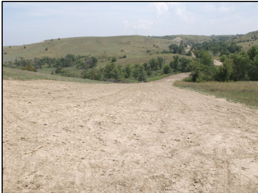
Photo 14. Direction: East. Depicted above is the pipeline corridor done the side of the hill previously mentioned. The corridor still needs to be seeded to fully complete remediation.
