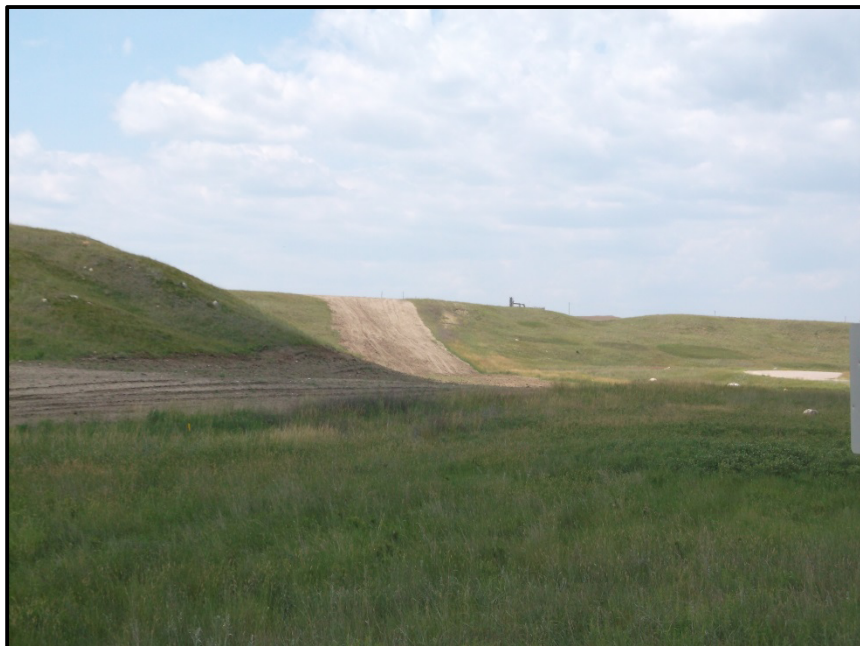
Photo 24. Direction: East. This portion of the corridor still needs to be seeded and monitored until fully reclaimed. It was apparent that the route corridor widths described in the application were used throughout the project as depicted in the picture above.
