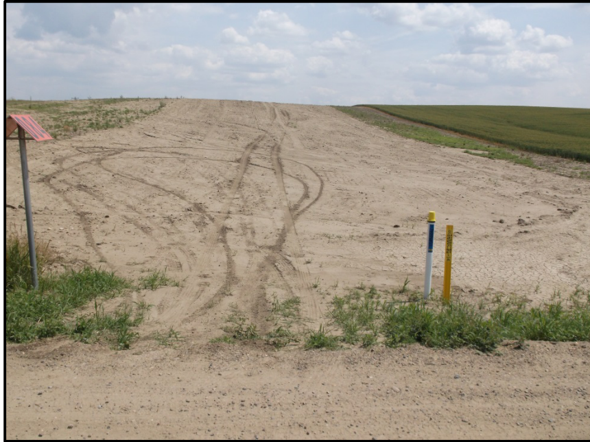
Photo 27. Direction: East. This is the section of the pipeline corridor that runs east and west parallel to 36 th St NW. The ROW along the road has not been completely reclaimed. Shown here is an access road crossing that was completed by boring underneath the road. Also shown is an above ground pipeline marker.
