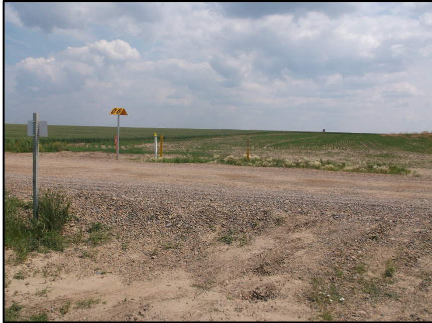
Photo 21. Direction: South. This is the bore location underneath 36 th St NW. No permanent impacts to the road were observed during the inspection. Above ground pipeline markers are also depicted in this photo.
