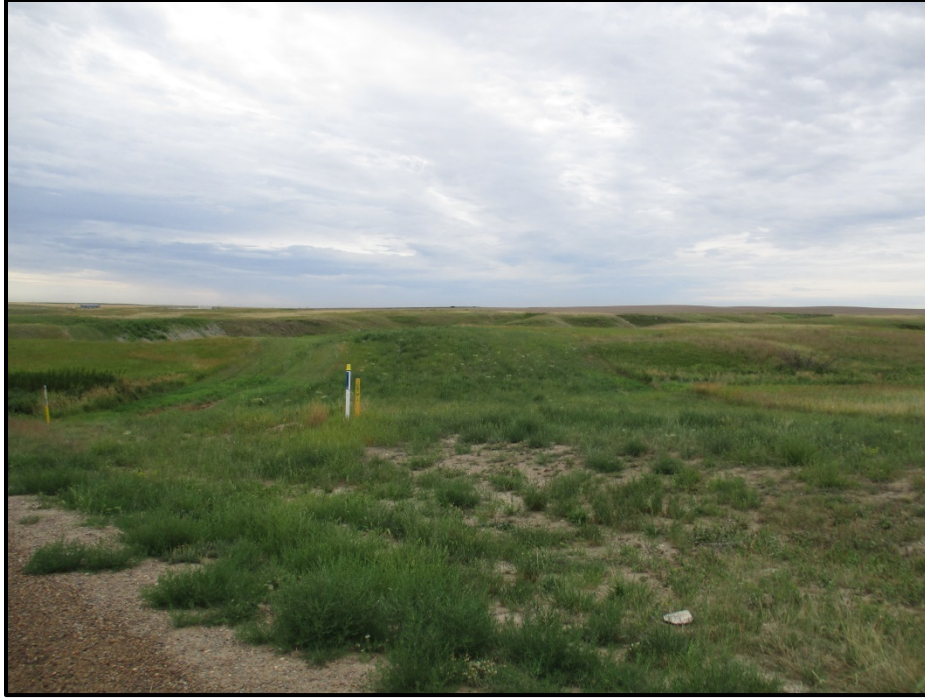
Photo 7. (GPS Point #7) - Pipeline ROW with pipeline markers, showing vegetation along a hilly area. Notice the light colored erosion control blanket on the hill in the background. Area was seeded in the fall of 2015 and the spring of 2016 and mowed in summer 2016. Direction looking southeast.
