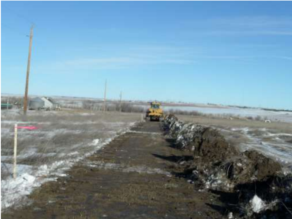
Report Photo #2 "Six (6) Inch Topsoil depth" at GPS Coordinates:
