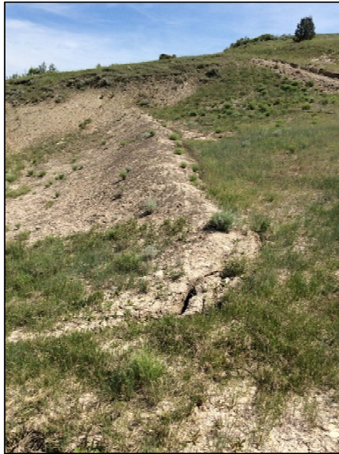
Photograph 5. Upper berm area. View to north
