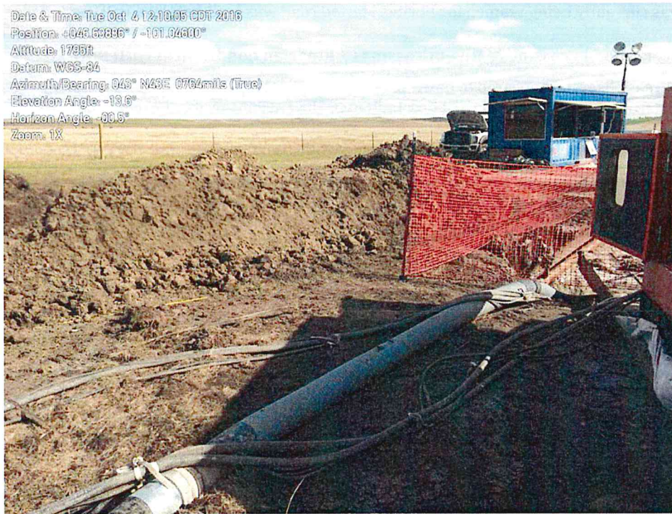
Report Photo #2 "Subsoils from HDD Bore Entry Pit on Unstripped Ground:
