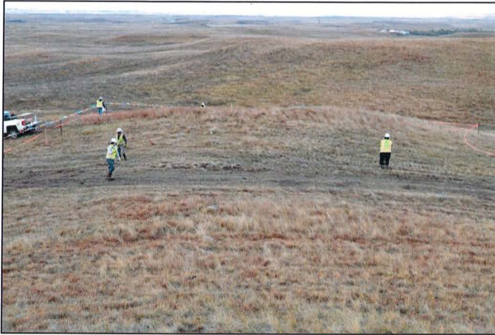
Figure 8. View of site with exclusionary flagging
