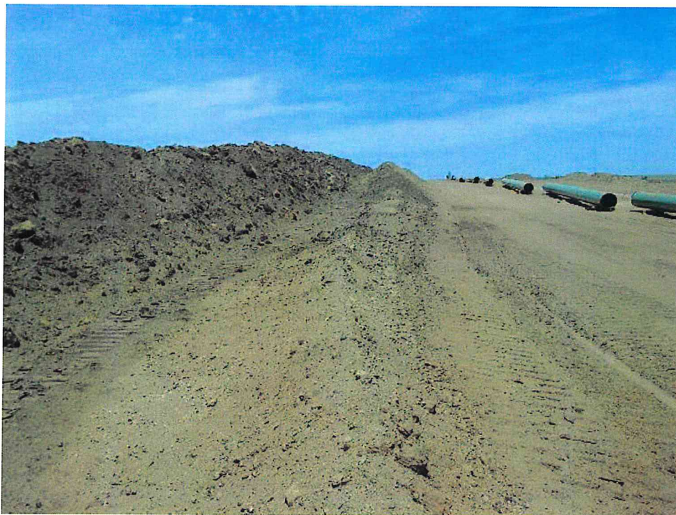
Report Photo #2 Topsoil-Subsoil Segregation at GPS Coordinates:
