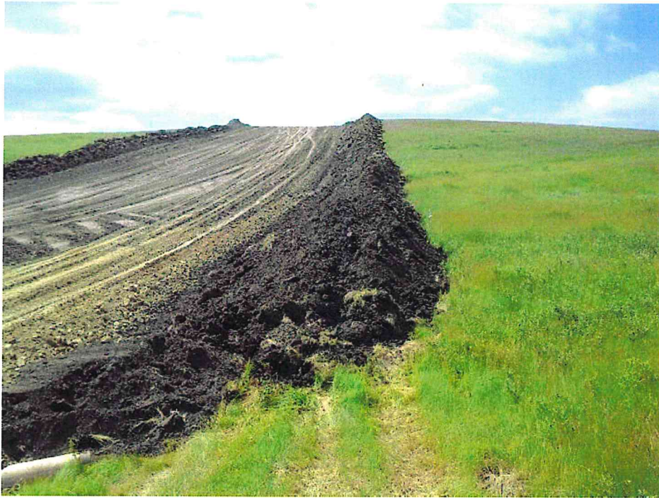
Report Photo #2 Subsoil piled on un-stripped ground at GPS Coordinates: 47.516944° N 102.835278° W
