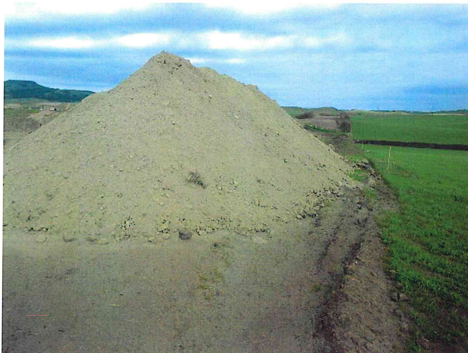
Report Photo #2 Subsoil piled on un-stripped ground at GPS Coordinates: 47.516944° N 102.835278° W
