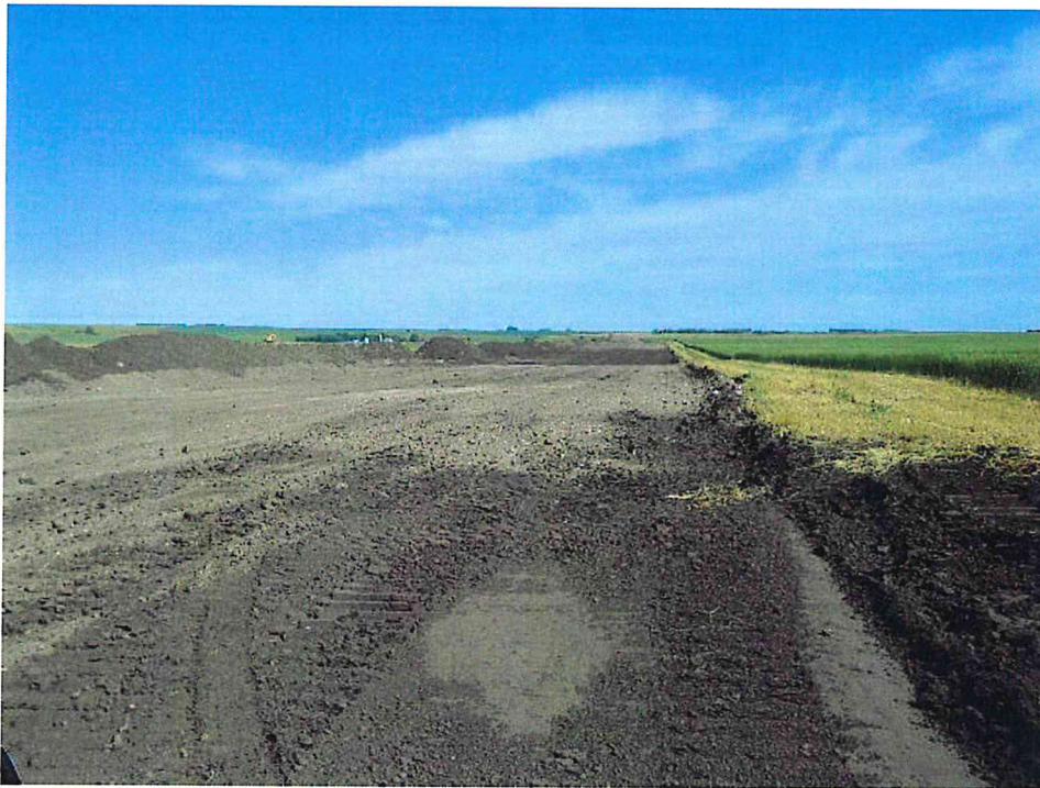
Report Photo #2 Topsoil-Subsoil Segregation at GPS Coordinates:
