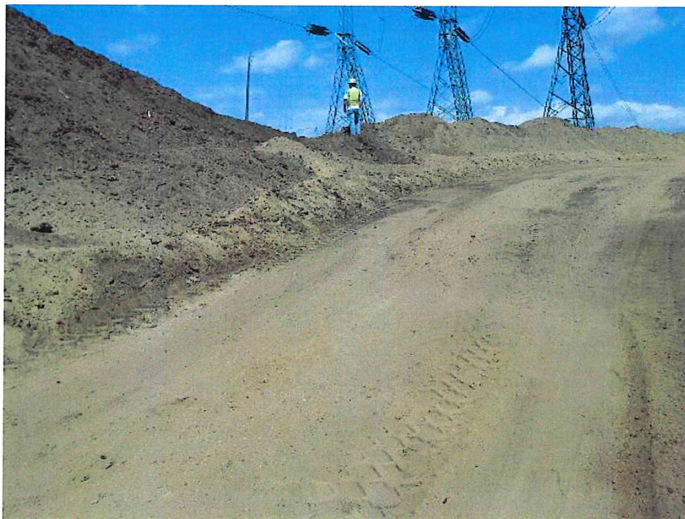
Report Photo #2 "Subsoil stacked against topsoil" at GPS Coordinates:
