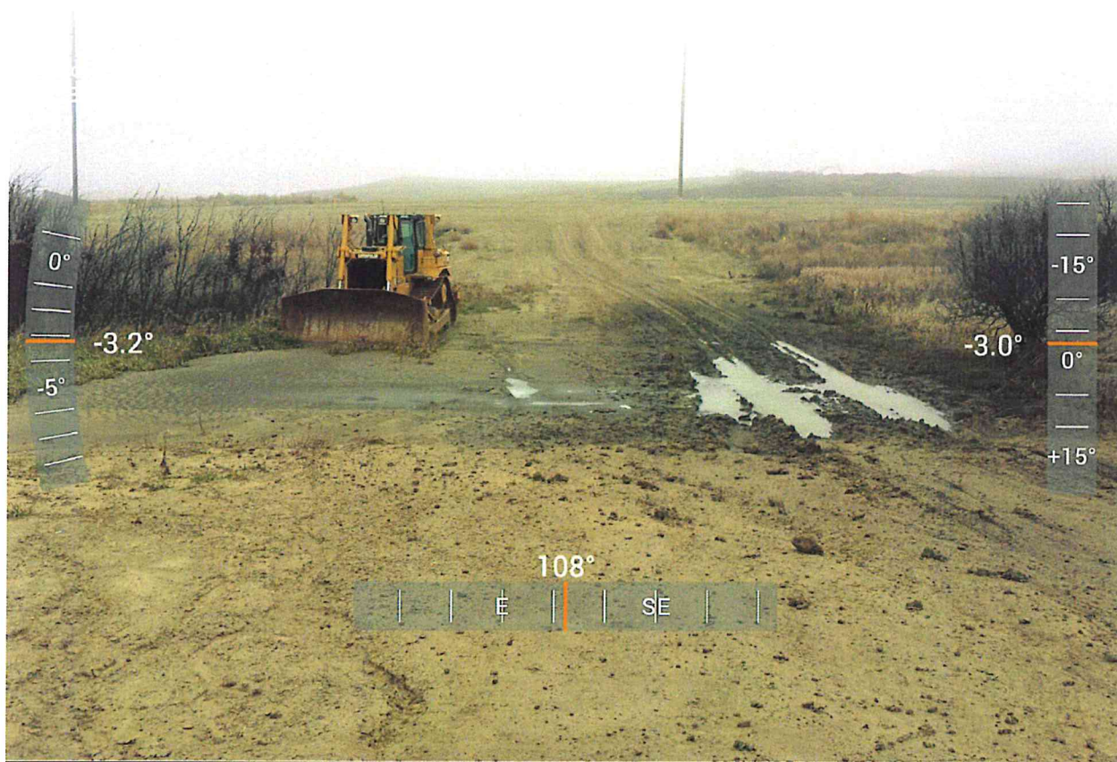
Photo 6 -Trees and shrubs removed at Johnson's Corner Terminal at 47.802597°N -102.928564°W.
