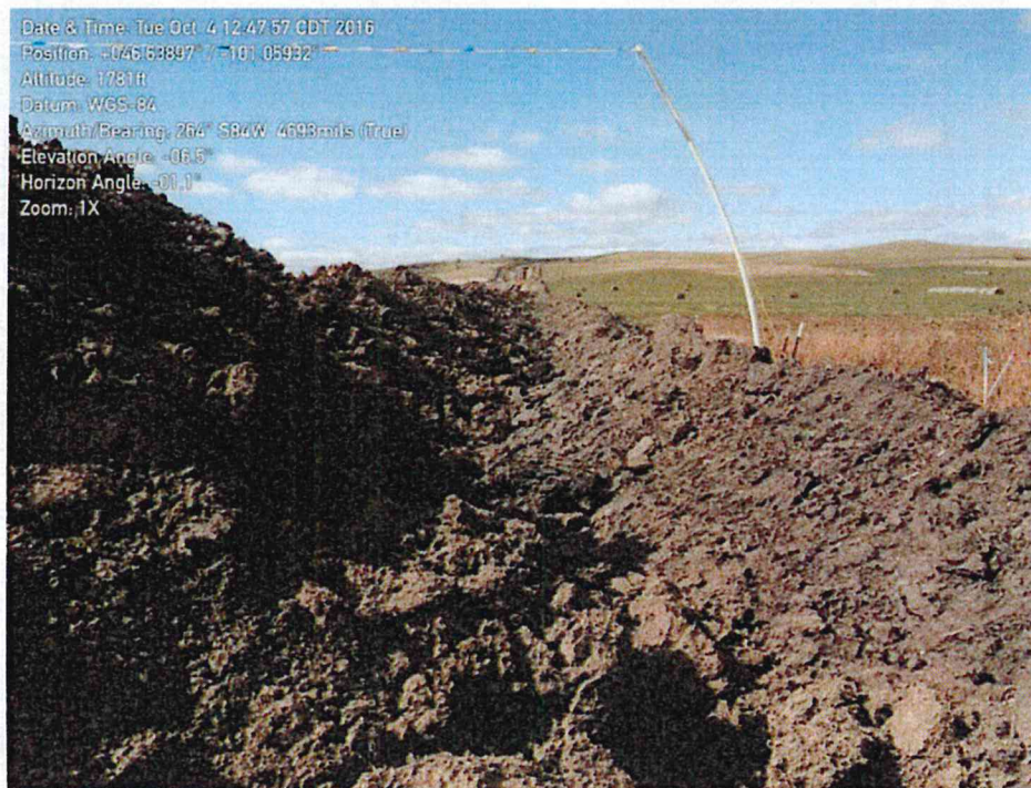
Report Photo #4 "Trench Subsoils Bordering/Overlapping with Topsoil Pile: 46.63897°N 101.05932°W
