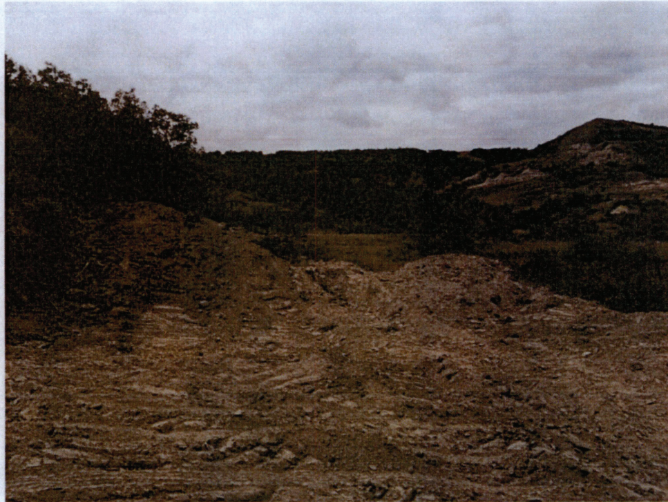
NOTE: Topsoil stacked on subsoil
