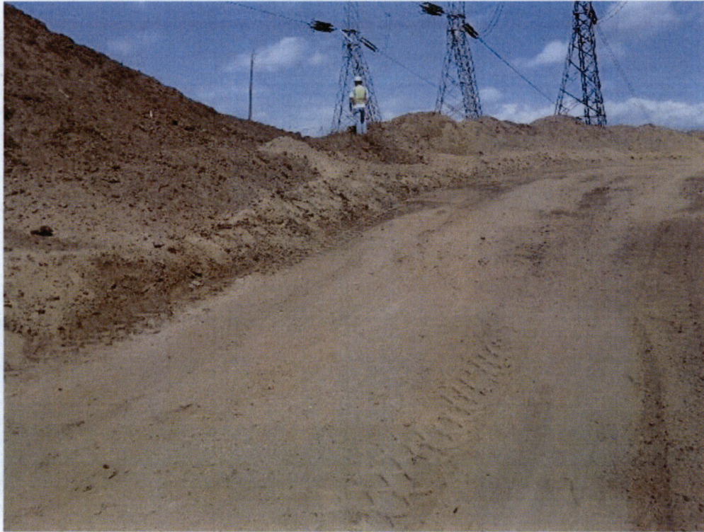
Report Photo #1 "Subsoil Mixing with Topsoil" at GPS Coordinates:
